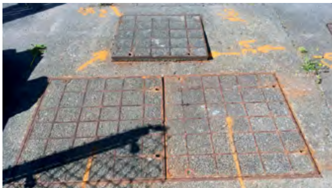
Covers were showing signs of severe corrosion
