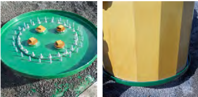
Fibrelite's 42" E85 compatible tank sumps being installed on double wall steel tanks
