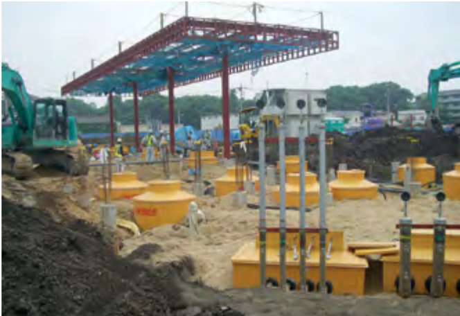
Site under construction
