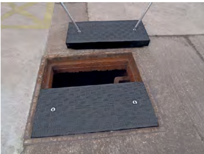
Bespoke Fibrelite covers installed into existing frame
