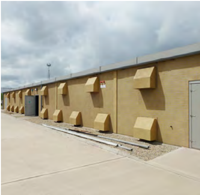
UK gas valve plant
