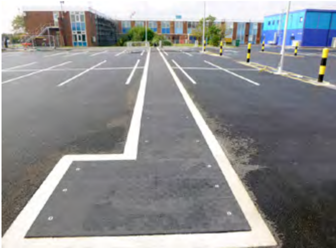
Lindley Oil Refinery, Killingholme, UK
