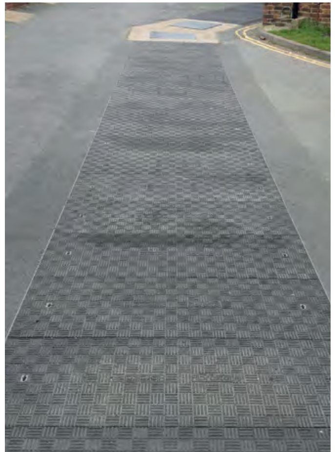
The same stretch following Fibrelite install
