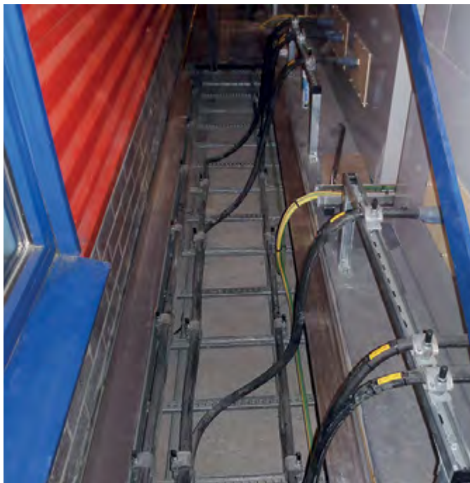
High and low voltage cables leaving trench to switchboard at regular intervals
