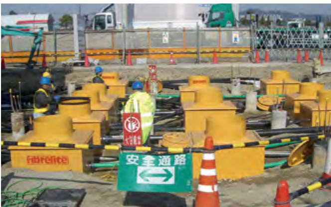
Vacuum tested tank sumps
