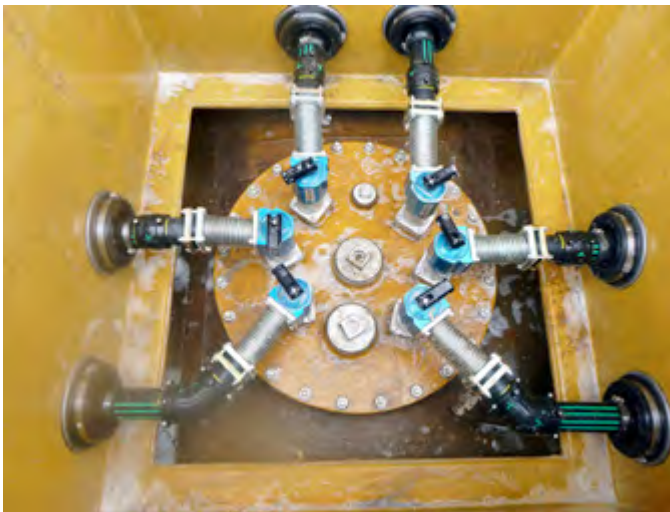
The Fibrelite site team conducted a vacuum test on site after the install
