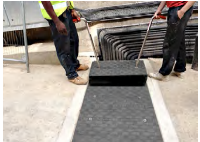
Fibrelite's ergonomically designed lifting handle make for easy and safe removal and entry to the ducting below
