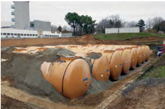
A demanding district heating redevelopment project in Rennes, France
