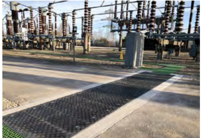
Fibrelite covers and frames were designed to fit existing apertures
