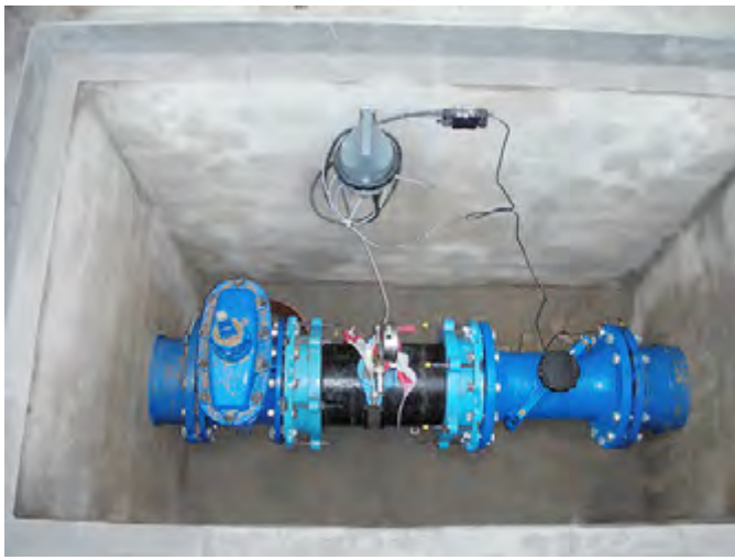
Underground water monitoring system (Image credit: Aguas de Cádiz)
