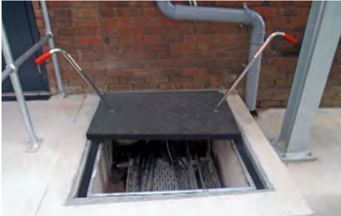
Sealed Fibrelite covers prevent water ingress
