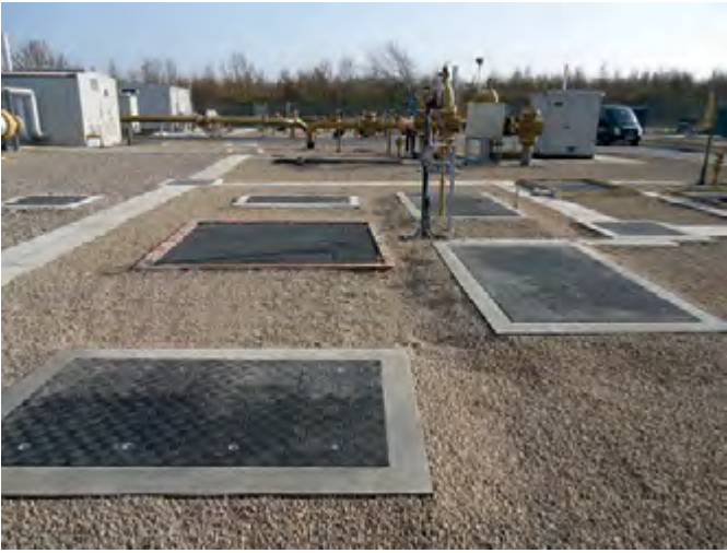
Corroded and damaged cast iron and concrete covers were replaced with Fibrelite's lightweight trench panels
