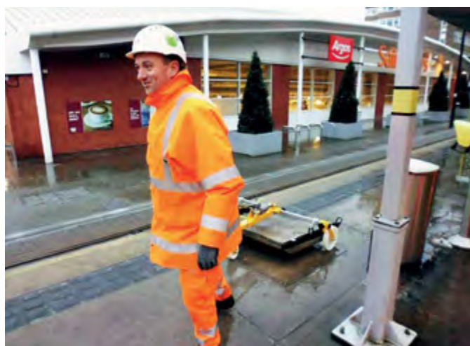
The previously installed heavy concrete covers
