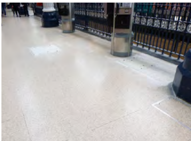
Fibrelite covers provide a safe walking surface for station users
