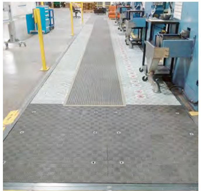
Lightweight Fibrelite FRP trench covers allow easy safe manual removal
