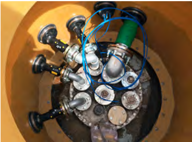
OPW provided a long-lasting containment system
