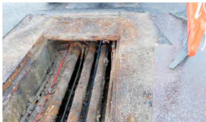
Previously installed failing concrete and metal covers
