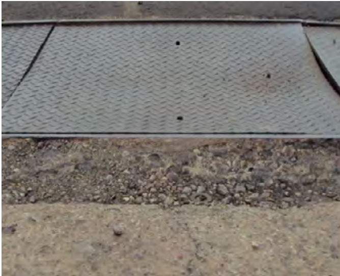
Corroded and deformed cheap steel covers
