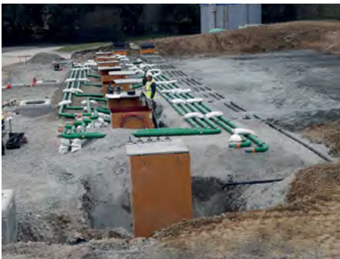
OPW provided a tailor-made KPS piping solution
