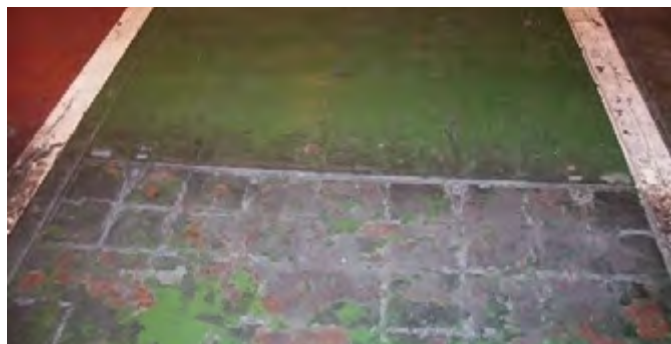
Once removed the concrete covers would never sit back in the frame correctly
