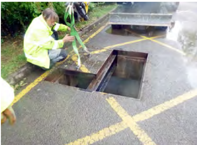
Due to the weight and difficulty in removing the covers critical time is lost in emergency situations
