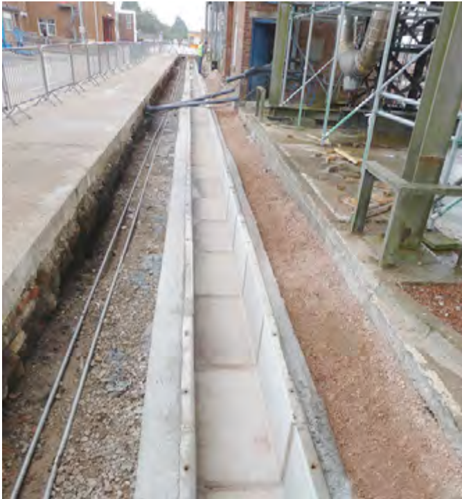
From an initial website search for lightweight composite panels to the installation of 190 new Fibrelite covers
