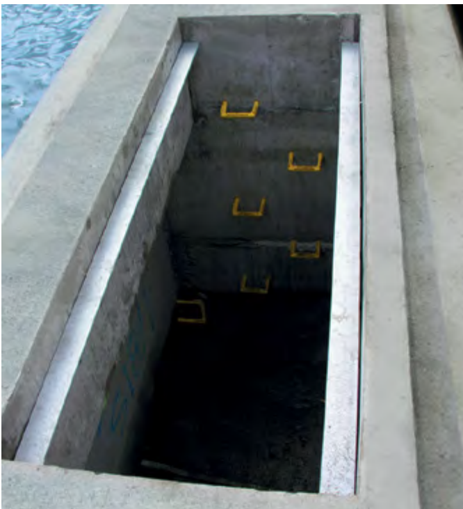
Access pit along edge of quay
