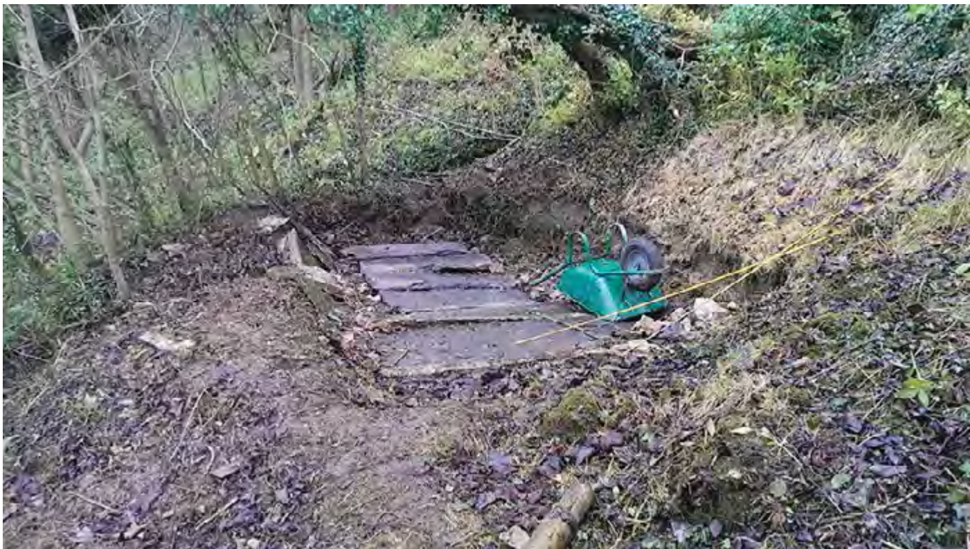
Old heavy slate covers posed a lifting hazard when access was required
