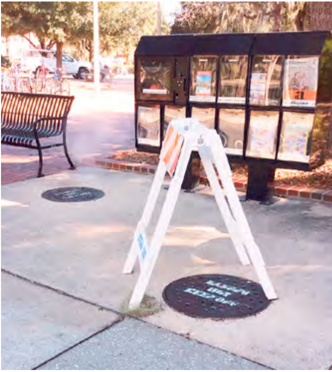
Original cast iron covers at the University were blocked because of their high temperatures due to steam.
