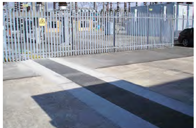
The EN 124 D400 tonne load tested lightweight covers
