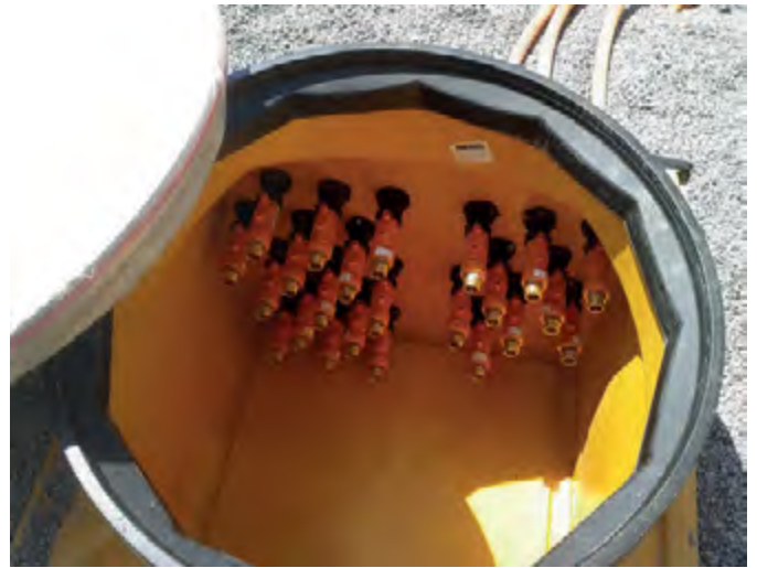
Cable drawpit with 32mm conduit piping
