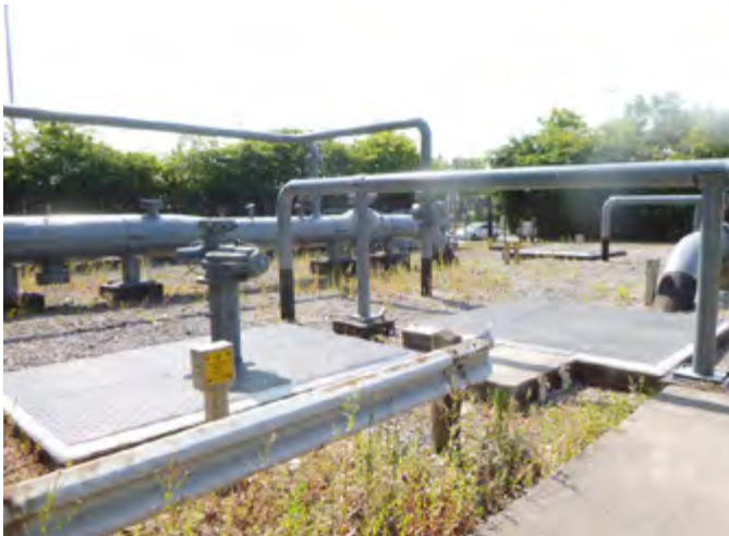
Cadent Gas Valve Pits, North West England
