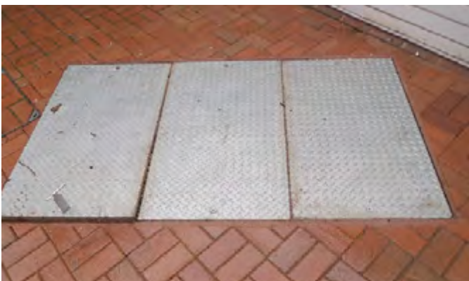
Previously installed odour-emitting galvanised covers
