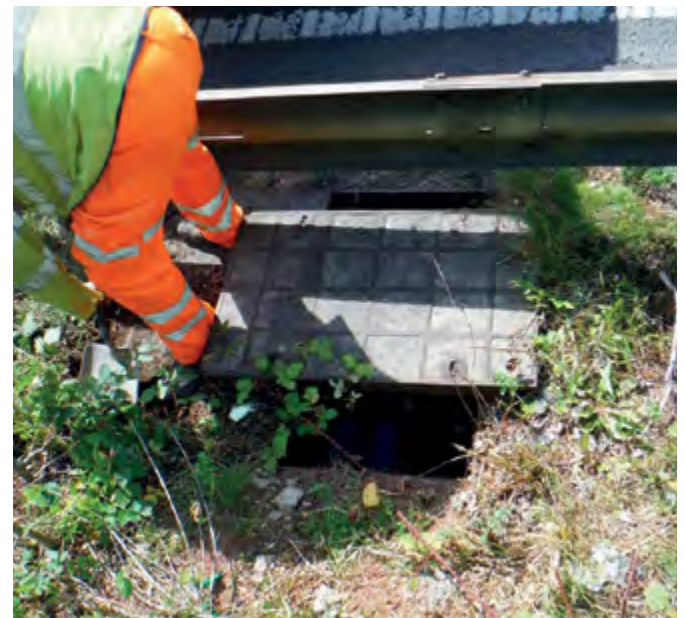
Damaged cast iron and concrete cover
