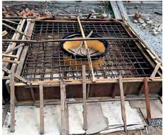
Prefabricating concrete plinth with Fibrelite FL90 frame
