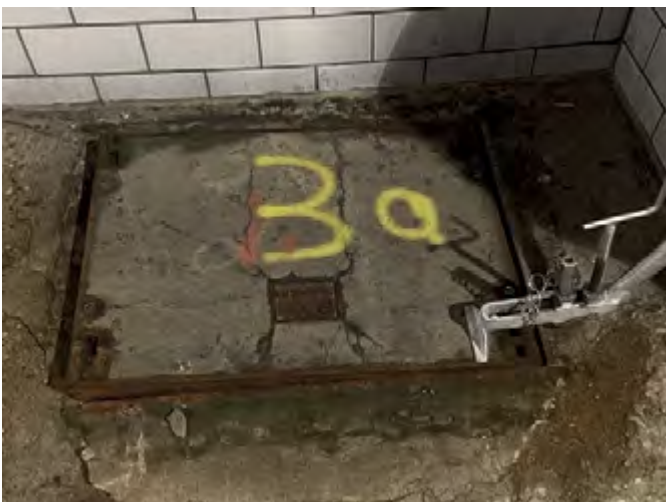
Old unsafe concrete covers
