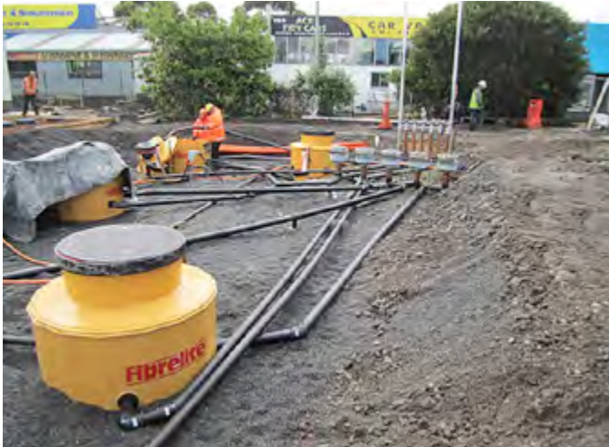
Fibrelite sumps are vacuum testable ensure watertightness
