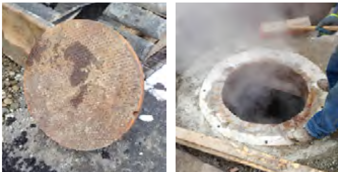
Large cast iron covers are both very heavy and extremely hot when exposed to steam within the manhole
