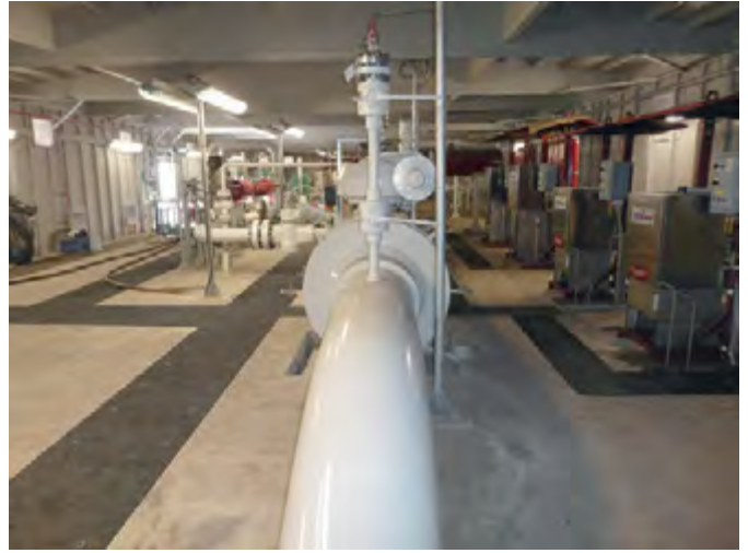
Longer length trenches with no additional support
