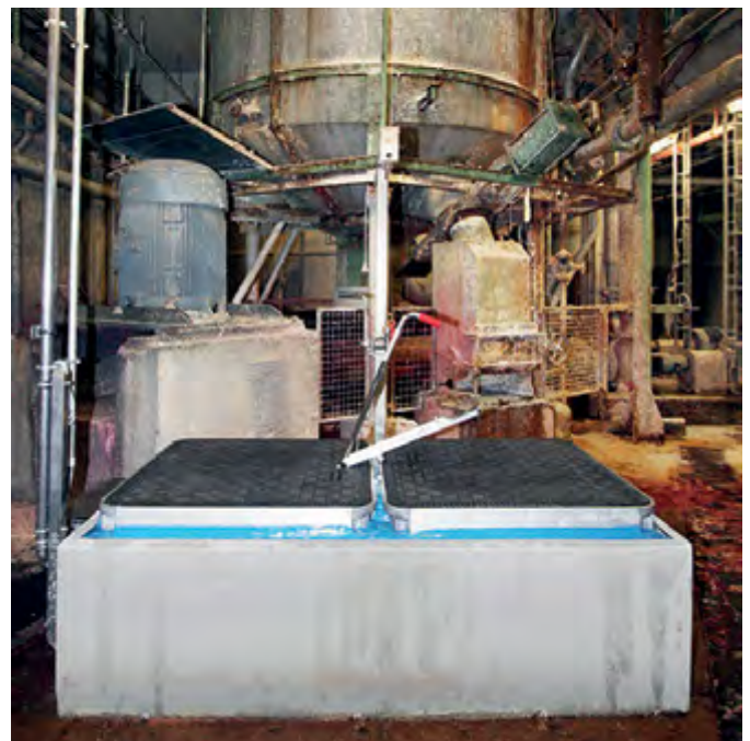
Complete installed Fibrelite covers
