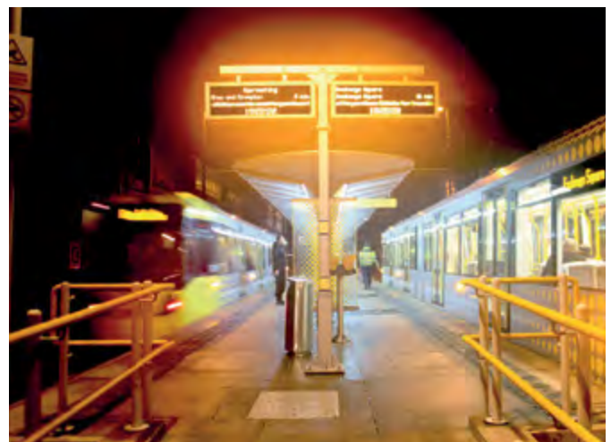
Fibrelite covers provide a safe walking surface in all weather conditions
