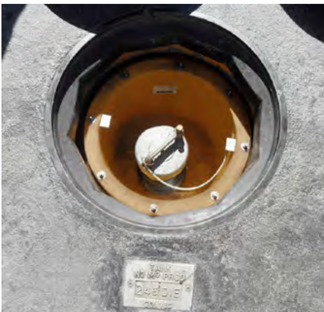
Fibrelite direct fill spill buckets (without drain back to tank) specified by Total
