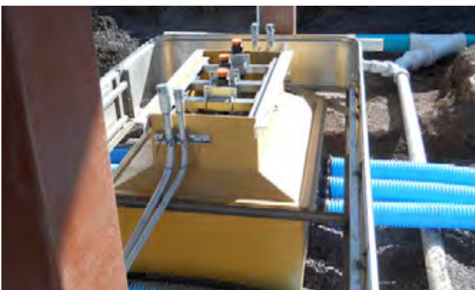
Fibrelite's E85 compatible Encore 500 dispenser sumps
