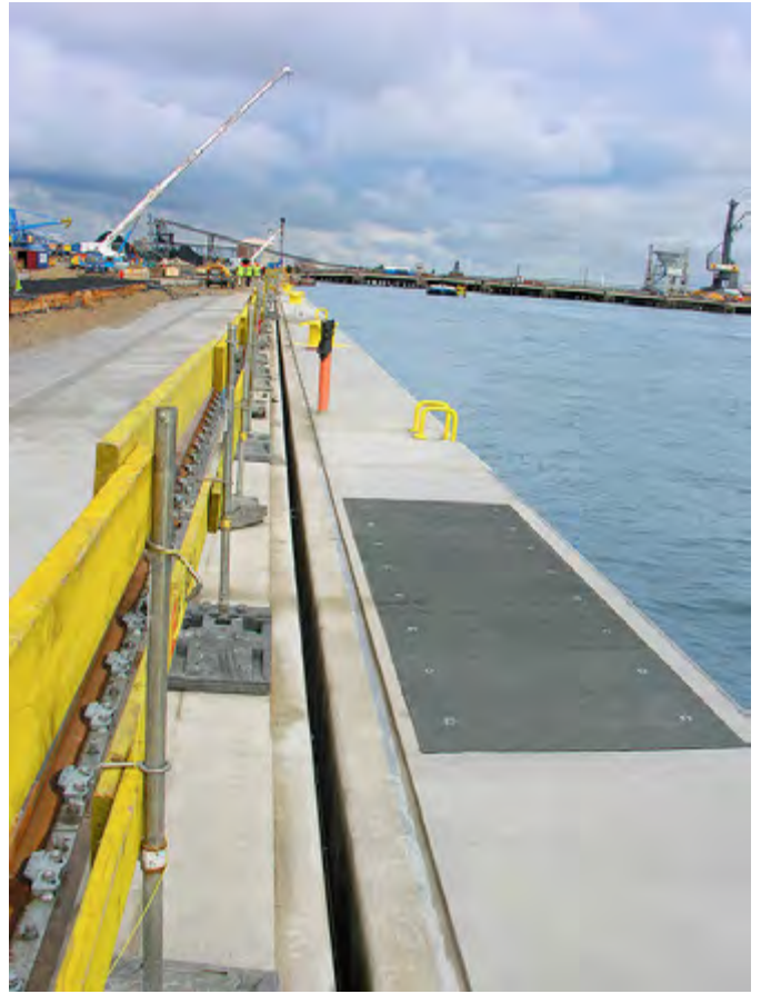
D400 load rated trench covers allowing safe manual removal
