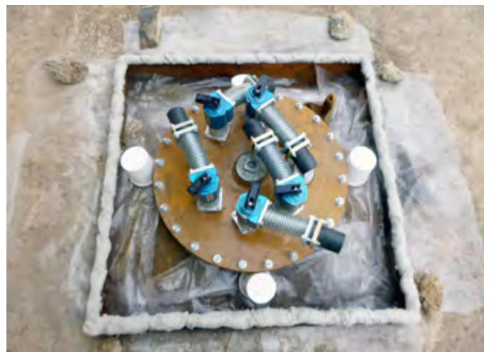
Preparation of surface for putty
