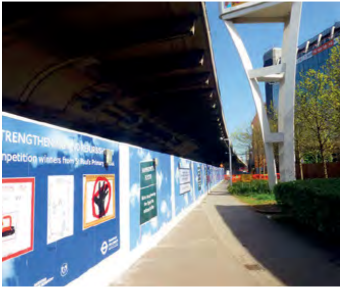
London Hammersmith flyover during refurbishment
