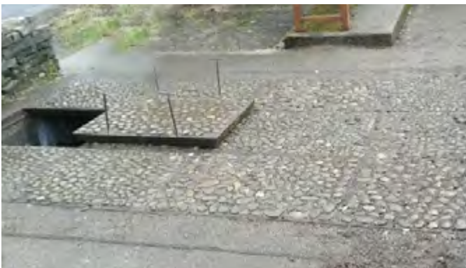
Cobbled covers requiring lifting equipment
