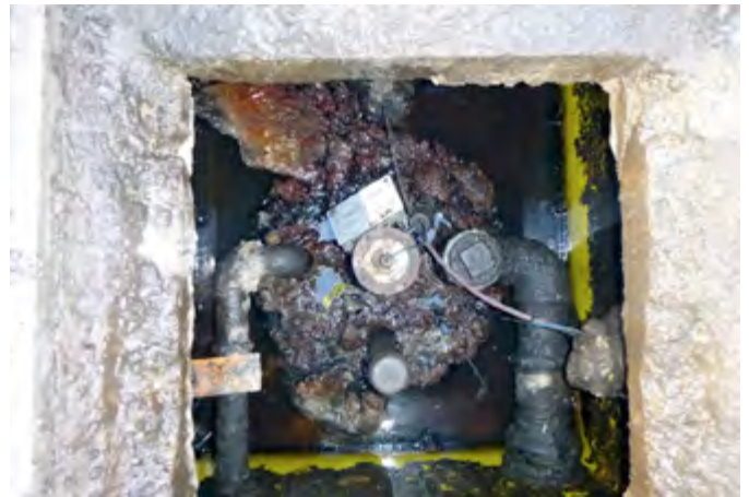
Shell required a retrofit watertight solution
