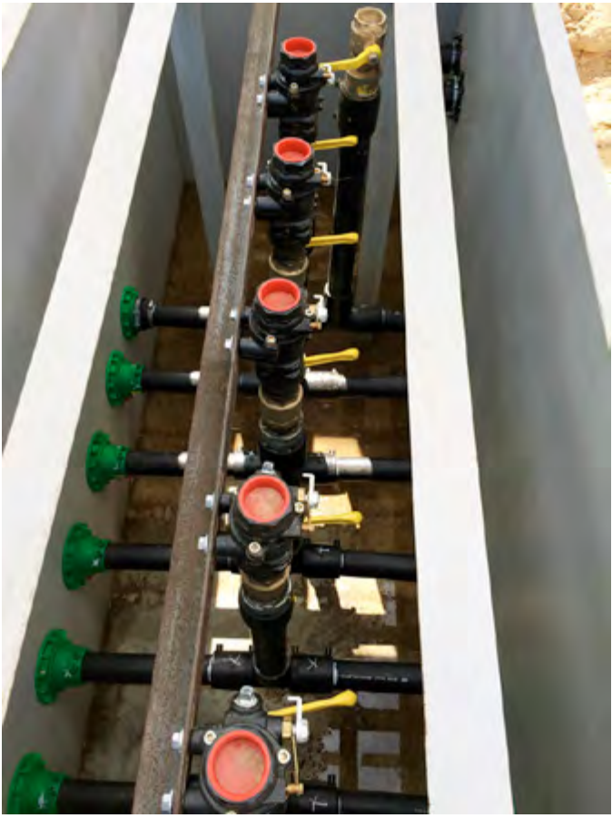
KPS piping combined with OPW shut-off valves creates a reliable fuelling solution
