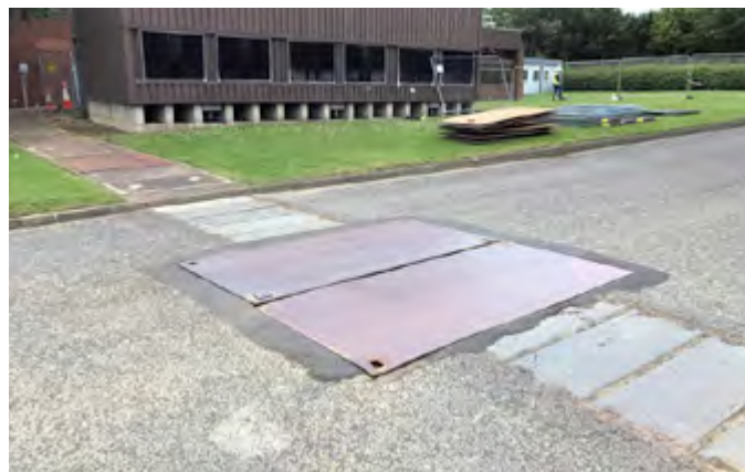
Sheets of metal had been installed as a temporary patch over failing concrete covers
