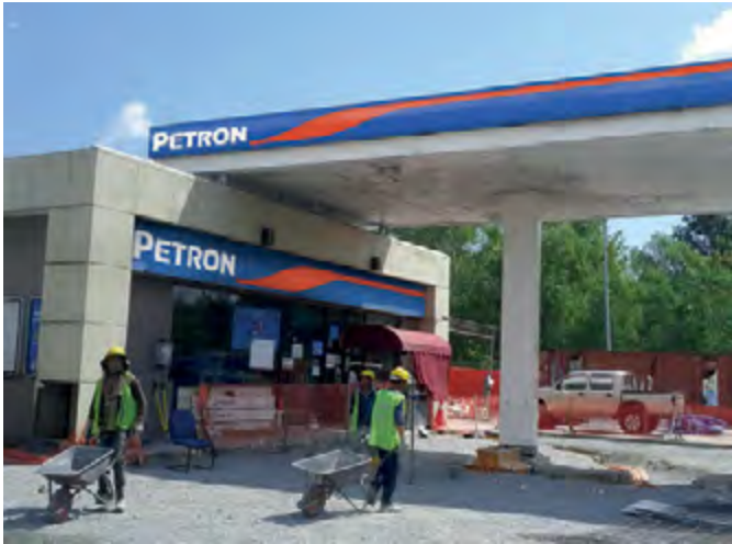
Site under construction
