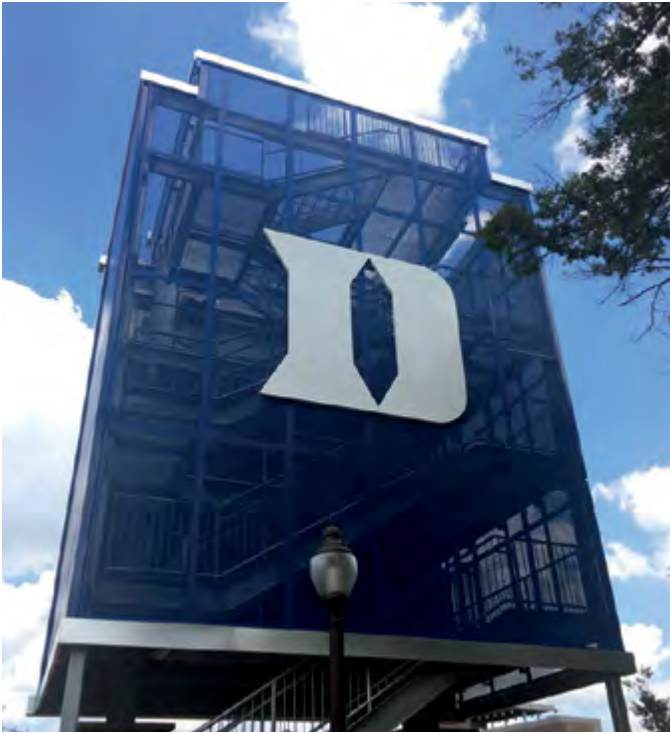
Duke University install Fibrelite trench covers
