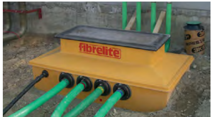
Fibrelite's vapour recovery transition sumps being vacuum tested to ensure a watertight installation
