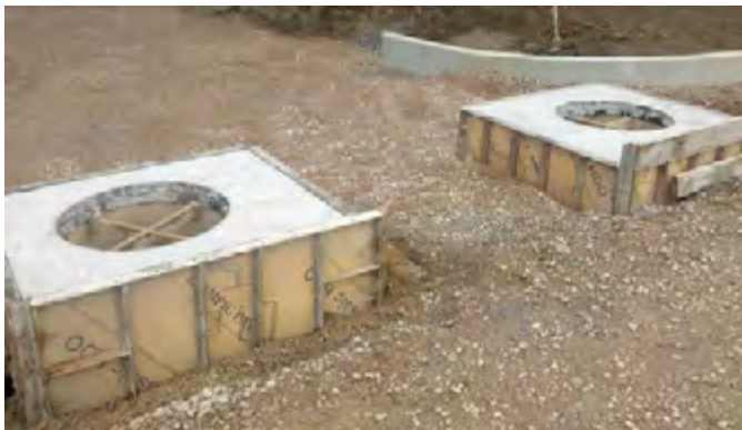
Pre-cast Fibrelite frames
