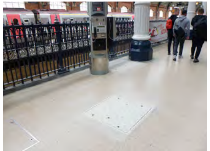
Fibrelite supplied covers which matched the base colour of the tiles
