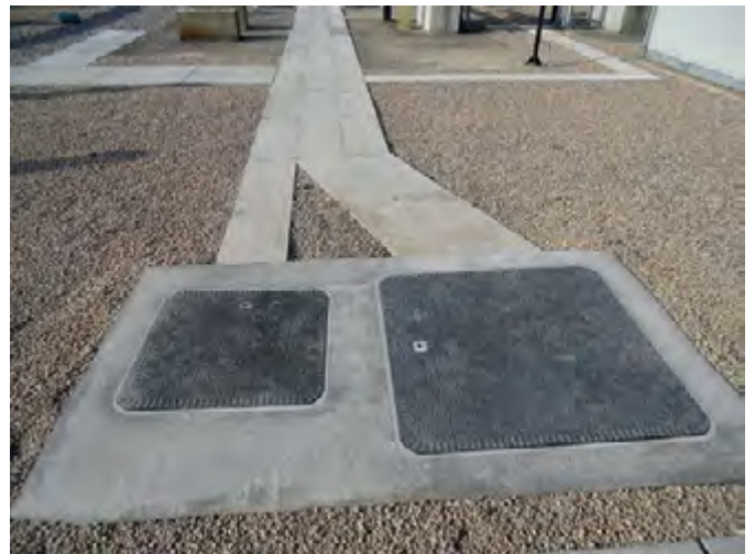
Fibrelite's watertight sealed manhole covers installed
