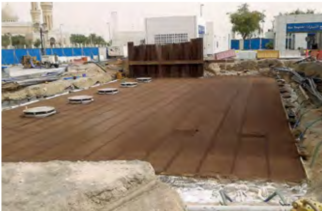
The deep installation required a robust corrosion resistant watertight solution
