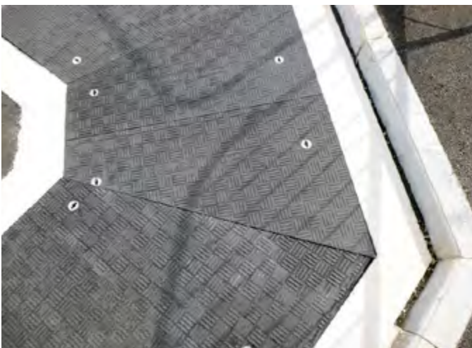
The skid resistant surface of Fibrelite covers removed the potential risk that would have been posed by concrete covers during periods of adverse weather or oil/chemical spillages
