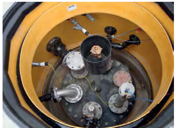
Fibrelite's 1.6m 12 sided tank sump with central dip stick
