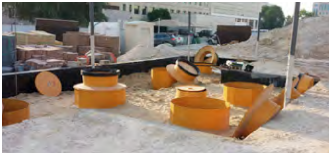
Fibrelite S14-390 tank sumps under installation
