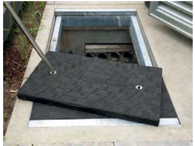
Fibrelite trench panels installed over the chamber
