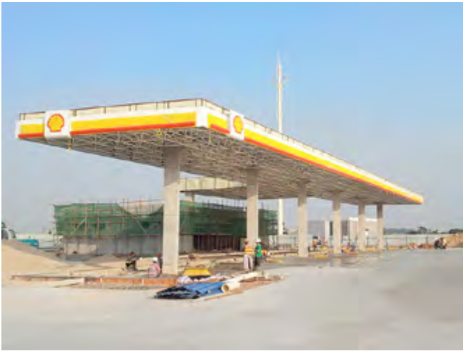
Site under construction
