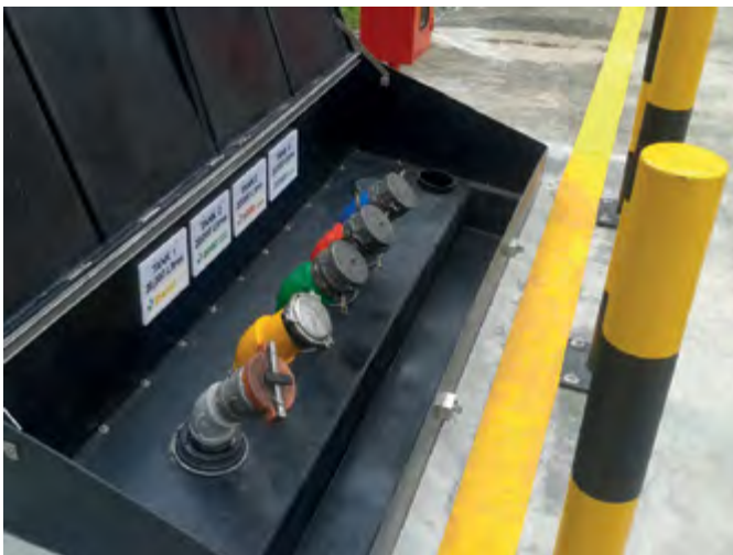
Fibrelite's S22SH-2/AGF above ground remote fill box
