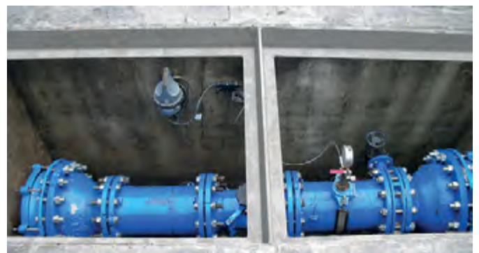
Fibrelite trench covers fitted into existing frames, preventing expensive breakouts and time for concrete to set (Image credit: Aguas de Cádiz)
