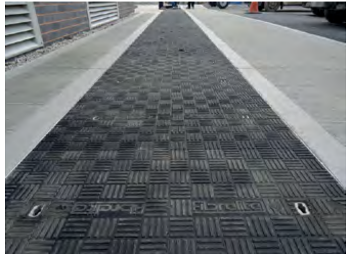
Fibrelite covers will not corrode or crumble like concrete or metal covers
