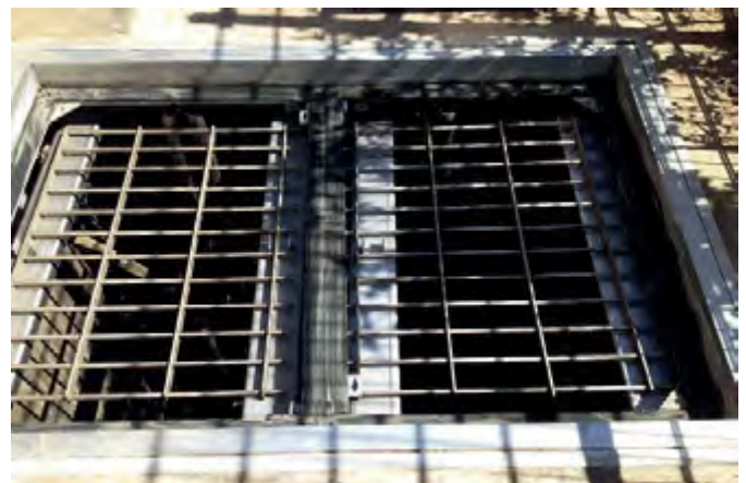
Removable beams hold safety grid
