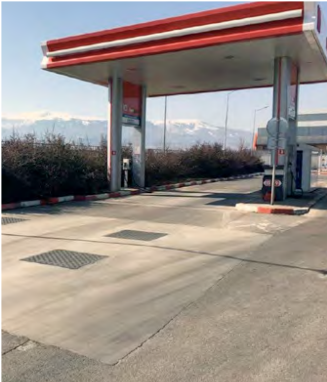
Fibrelite covers installed at a number of LUKOIL sites to replace failing cast iron covers
