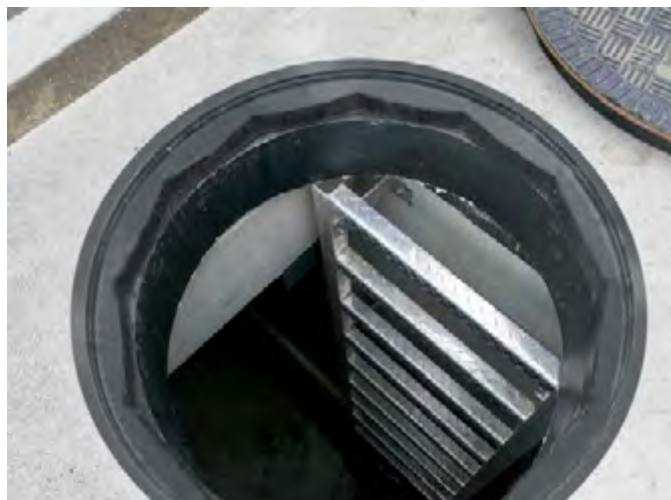
View from over the manhole
