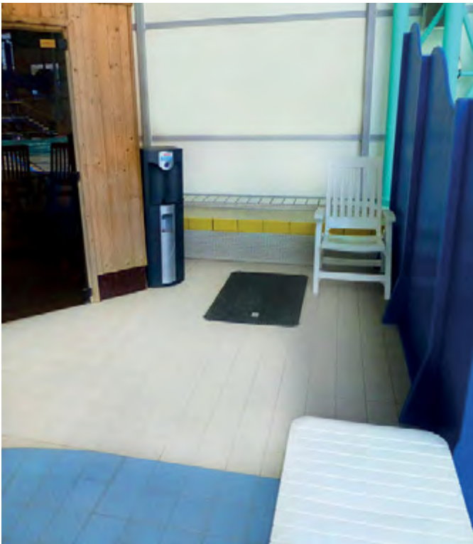
Leisure centres are highly corrosive environments with moisture and chlorine, making composites an obvious choice
