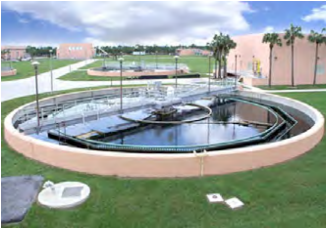
Concrete to Composites
