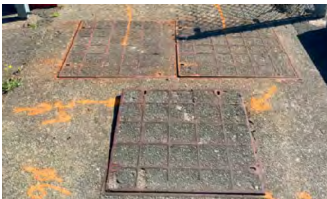
Previously installed heavy concrete recess covers
