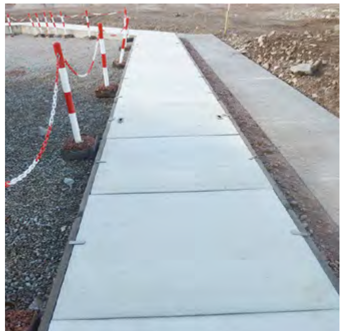
Concrete covers unable to withstand pedestrian traffic
