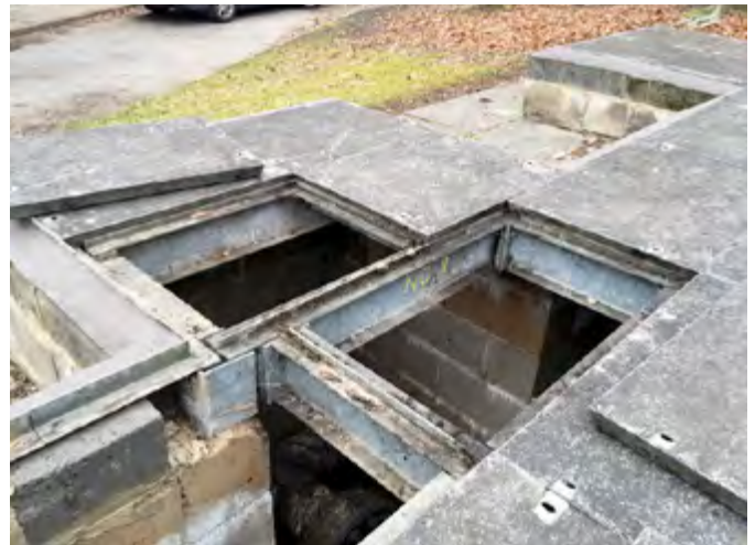
The previously installed obtrusive framework made access difficult and led to health and safety risks
