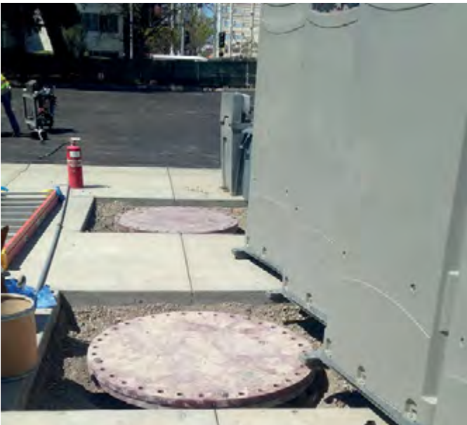
Fire manway lids (tank buried underneath)
