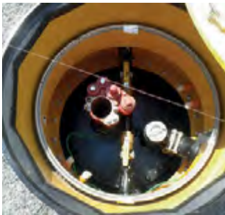
Fibrelite's 1.2m 16 sided turbine sumps being installed
