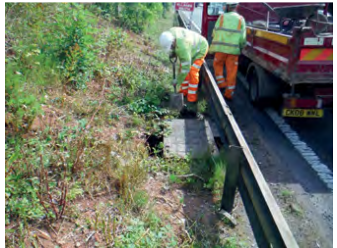
Heavy covers present a hazard for operators
