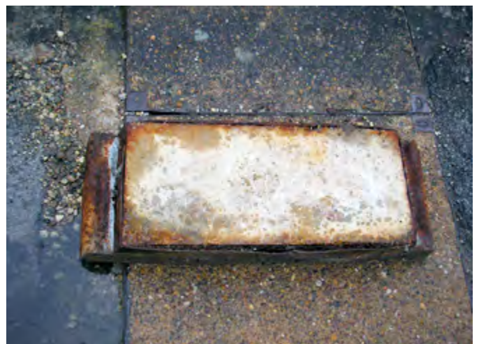
Corroded previously installed cover hinge
