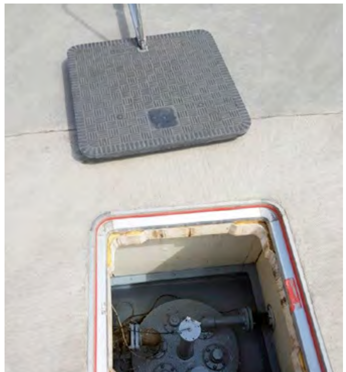
Lightweight new Fibrelite FL76 covers installed in Bulgaria for LUKOIL
