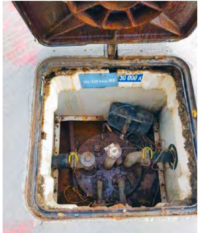
The previously installed cast iron manhole covers had rusted allowing water ingress
