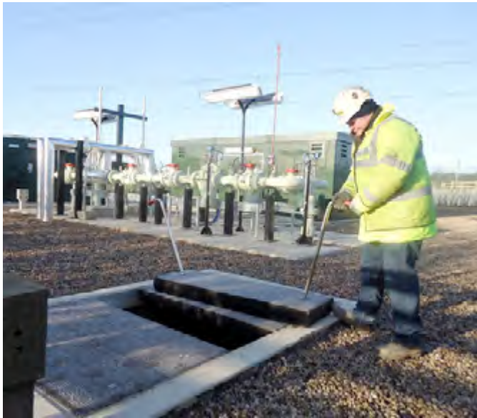
Easy and safe access to underground systems
