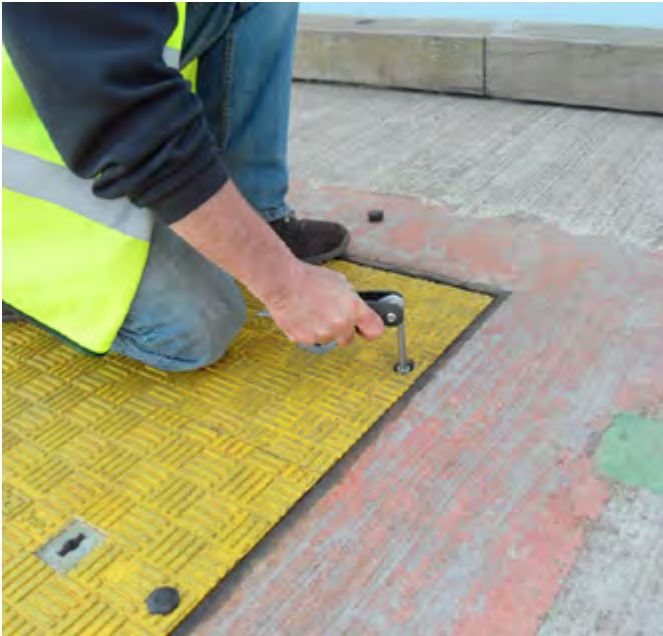
Operator removing the Fibrelite securing system
