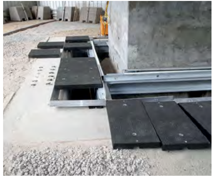
Bespoke composite trench covers designed with encapsulating frames
