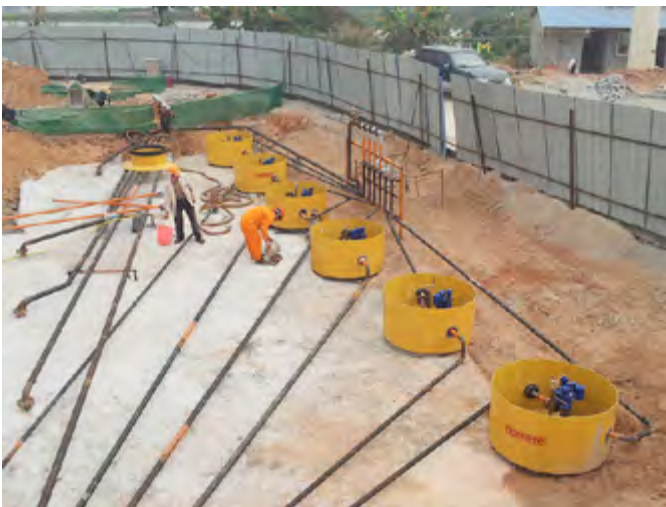
Fibrelite tank sumps (S14-390) being installed
