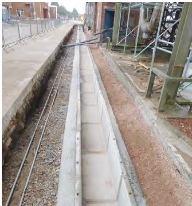
From an initial website search for lightweight composite panels to the installation of 190 new Fibrelite covers
