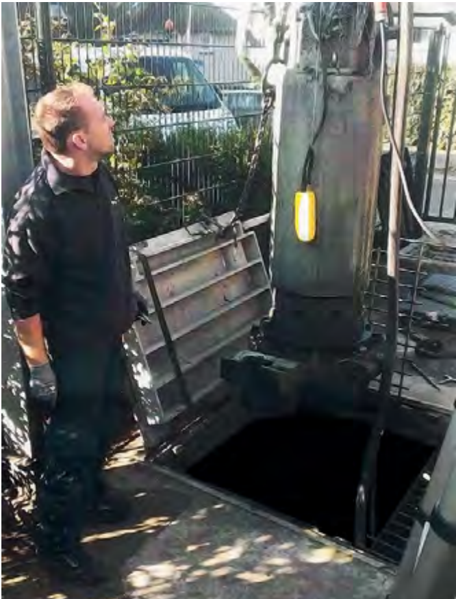
Heavy metal covers requiring 2 men and a crowbar to remove, emanating odours
