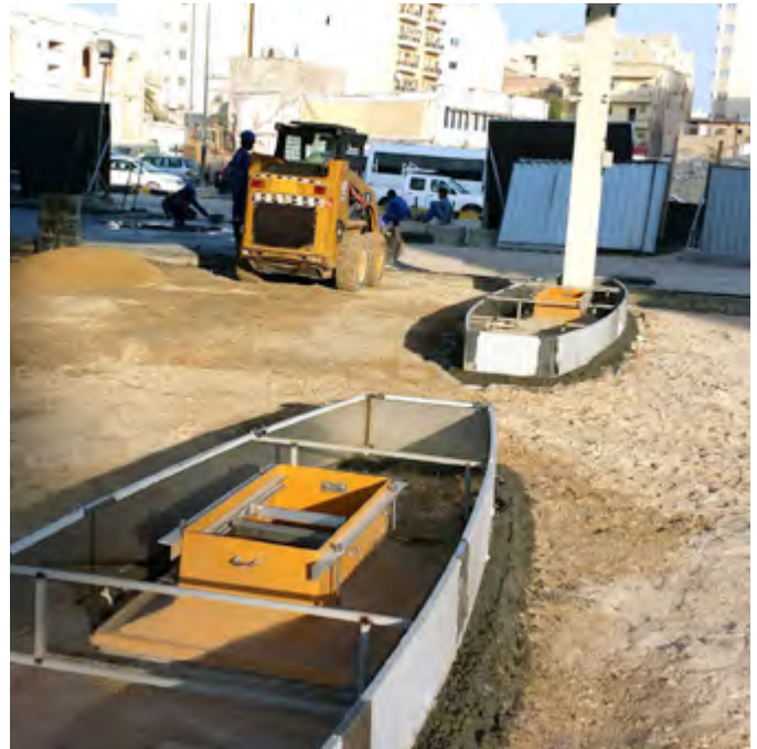
Fibrelite EL-G-E500 dispenser sumps ready for concreting
