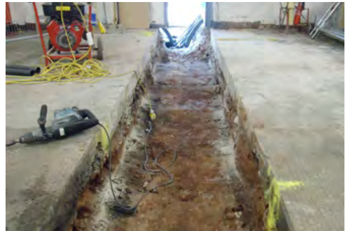
The trenches before Fibrelite install
