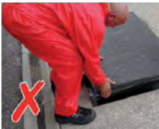
Dangerous lifting technique without Fibrelite lifting aid
