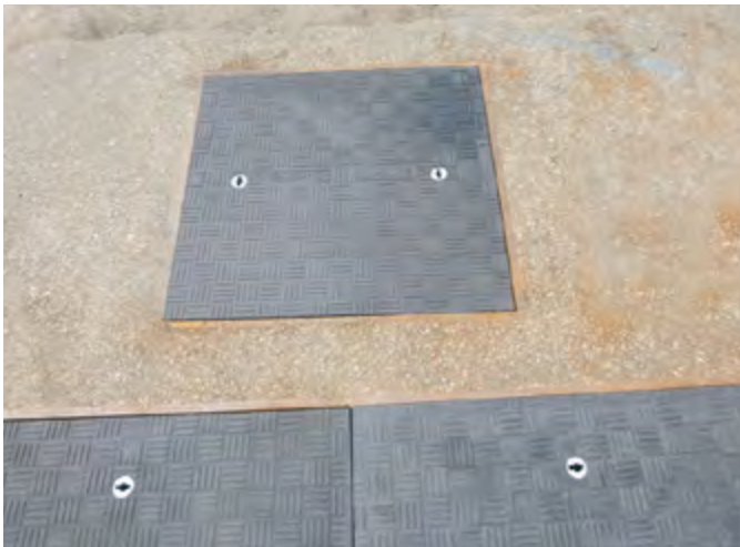
Covers were manufactured to fit existing frames
