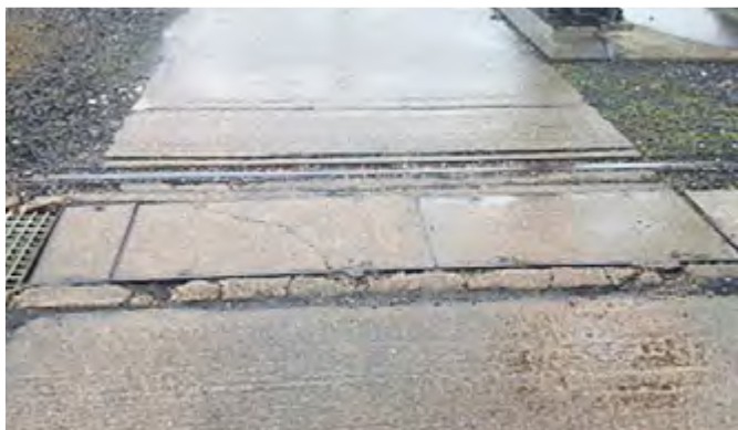
The previously installed cast iron frame showing signs of damage and corrosion
