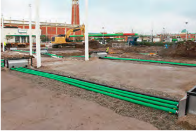
10m lengths of custom 75/63mm KPS straight pipe allowed fast installation without the need for a welding socket in middle
