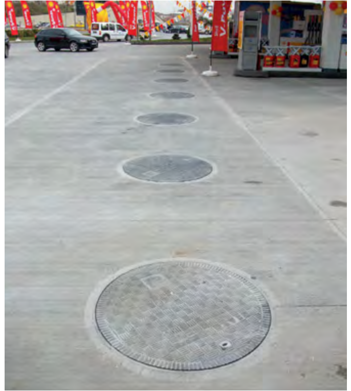
Fibrelite composite covers prevent surface water ingress into chambers
