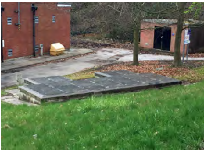
RJ Utilities required trench covers that would improve the efficiency and safety of the site
