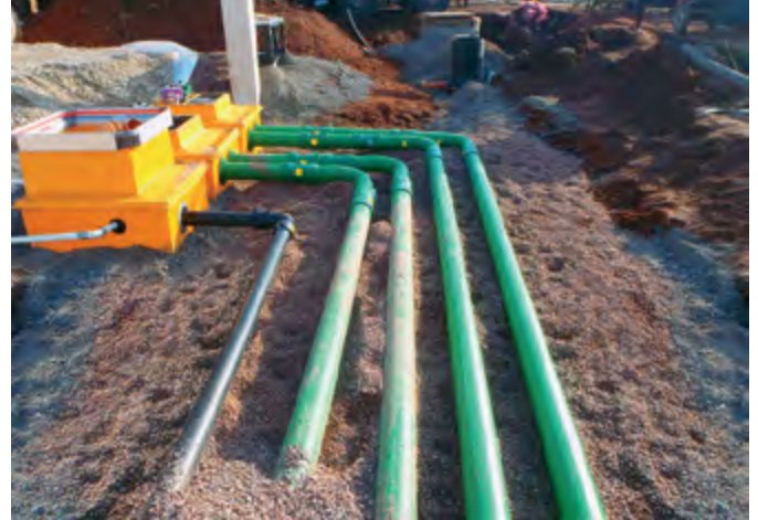
All integrated KPS fittings weld both pipe walls simultaneously
