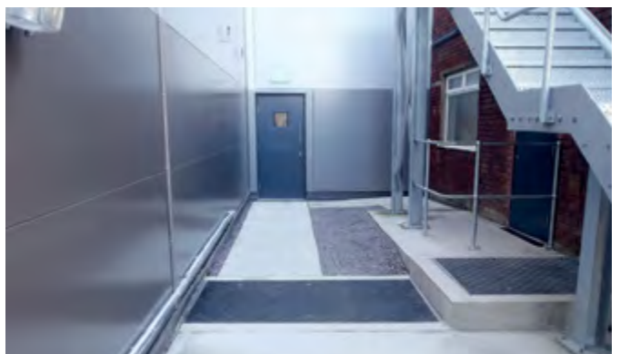
Retrofitted sealed Fibrelite covers installed
