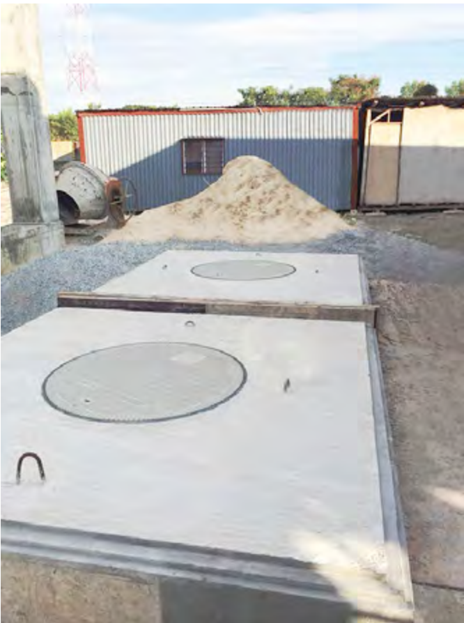
Plinths ready for installation
