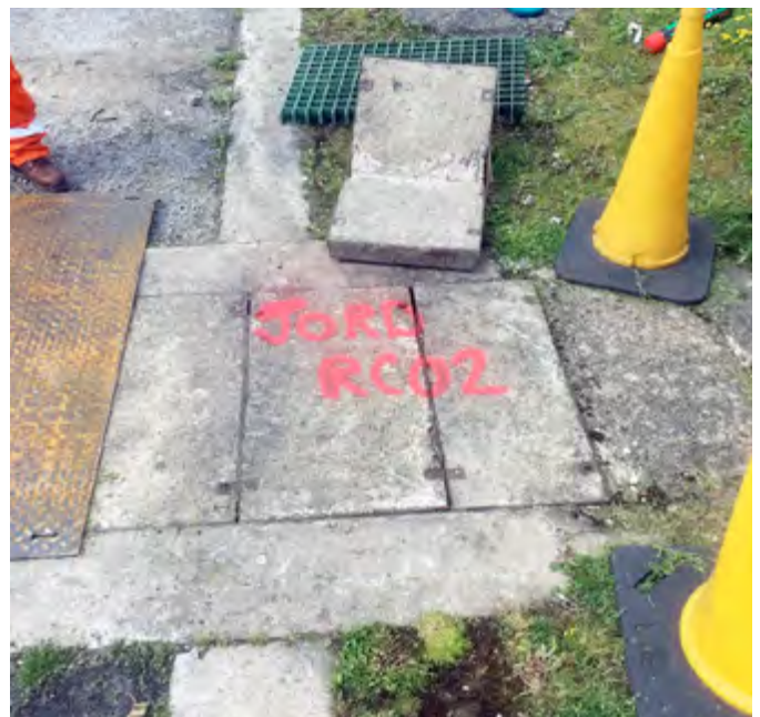
Covers were extremely heavy to lift
