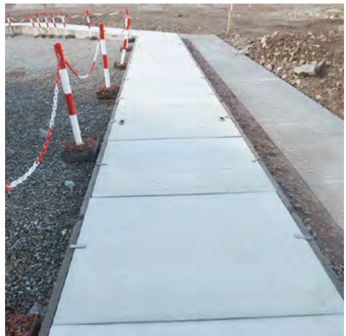
Concrete covers unable to withstand pedestrian traffic
