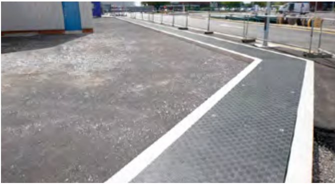
Fibrelite covers are chemically inert
