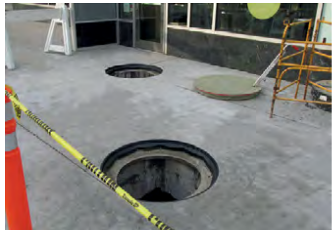
Fibrelite F95 composite cover installed in frame
