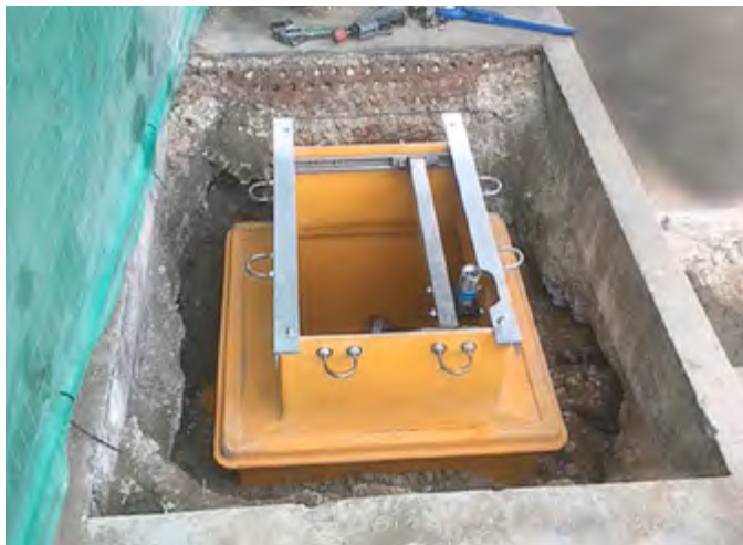
BP required retrofit chamber systems
