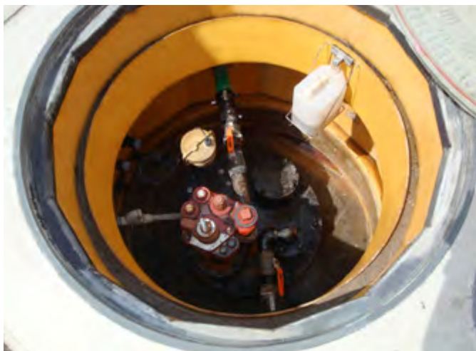
Fiberglass turbine sump with 55" tank collar
