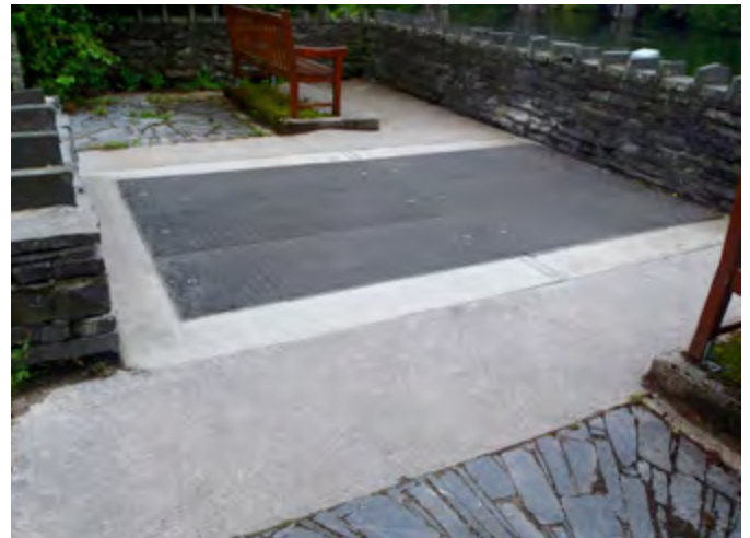
Lightweight Fibrelite trench covers now installed
