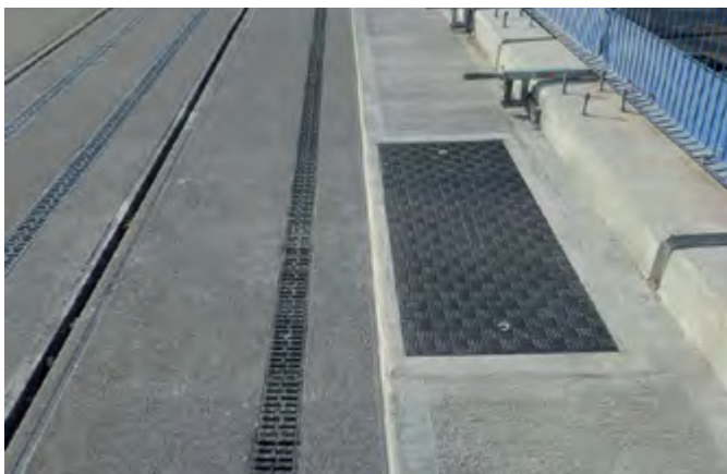
Bespoke trench covers for trackside gear
