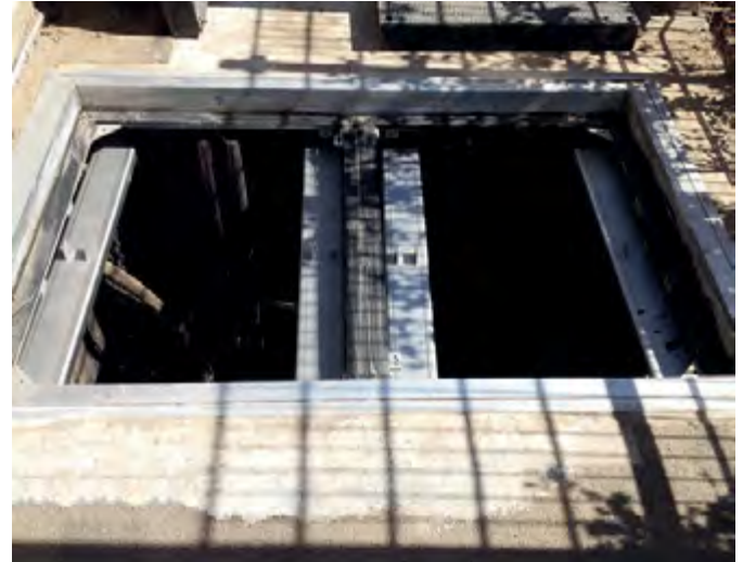
Removable centre beam supports covers
