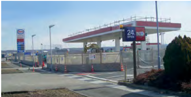
Site under construction
