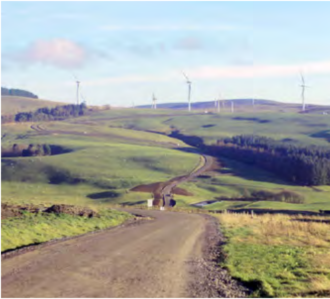
Garreg Lwyd wind farm under construction
