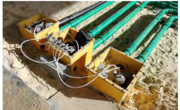
Secondarily contained Fibrelite remote fill sumps
