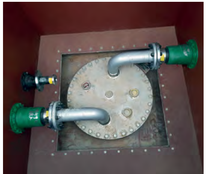
Fibrelite vent transition sump provided easy access to KPS single wall suction system and double wall suction system (pictured)
