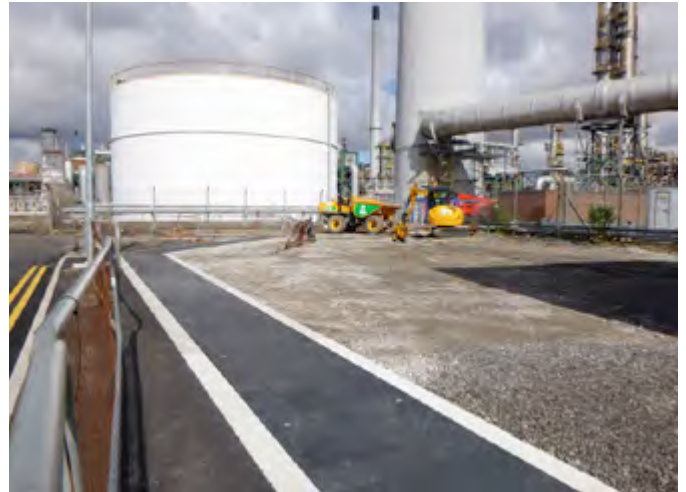
Fibrelite covers have resistance to extremely high temperatures and so can withstand the emissions from the steam pipes below them
