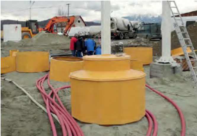
Gazprom have specified Fibrelite's fully conductive 1.6m dia chambers (S16) to facilitate easy maintenance post installation
