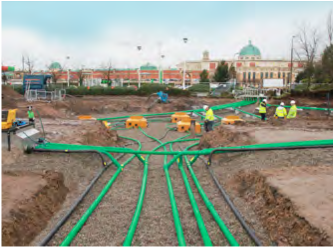
North England site under construction
