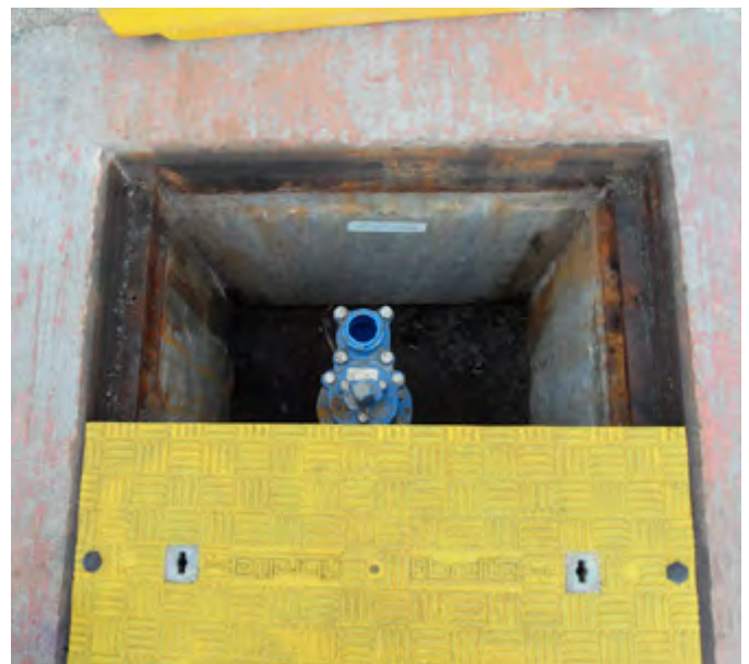
Previously both of the extremely heavy steel covers had to be removed to expose the isolation valve for the drinking water supply. Now only one Fibrelite trench cover needs to be removed
