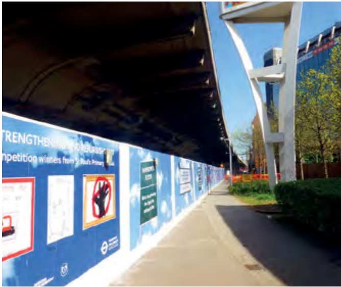
London Hammersmith flyover during refurbishment
