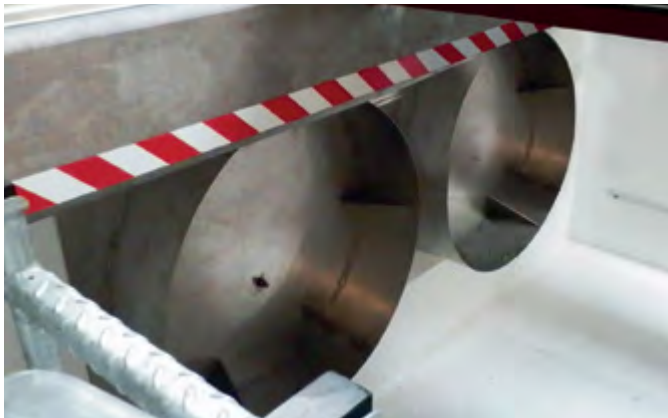
Underground pit to house crane supply lines
