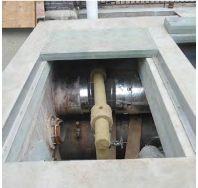
Six Fibrelite FM45 4' 6" (1.6m) wide anti-slip GRP composite trench panels being installed in the sidewalk
