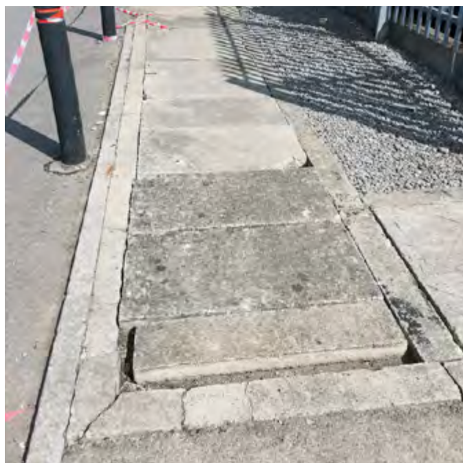
Previously installed failing concrete trench access covers
