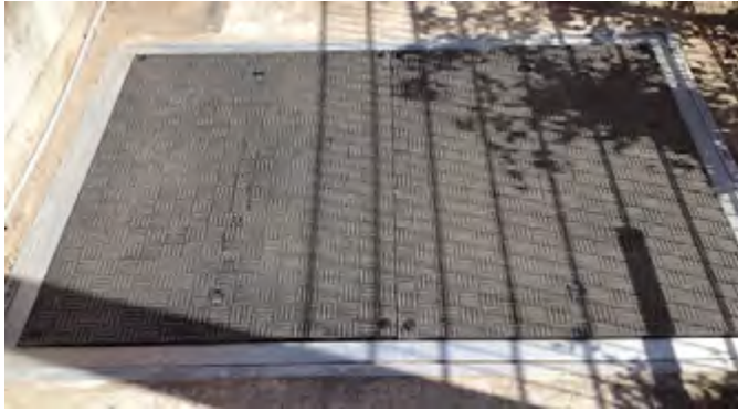
Sealed odour-tight covers installed
