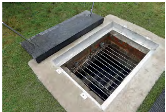
Safe and easy manual removal: Fibrelite FM45 covers are removed by hand from the CSOS (Combined Sewage Overflow System) chamber
