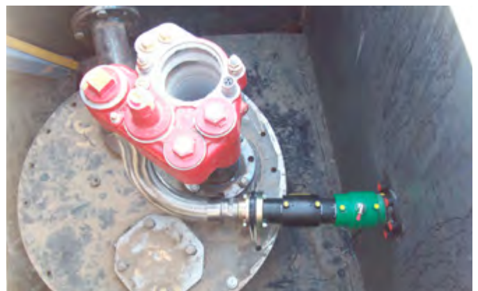
The KPS compact solution allowed for emergency valves to be installed under dispensers
