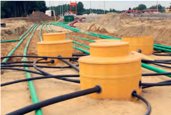
OPW continue to supply major oil company with filling station equipment
