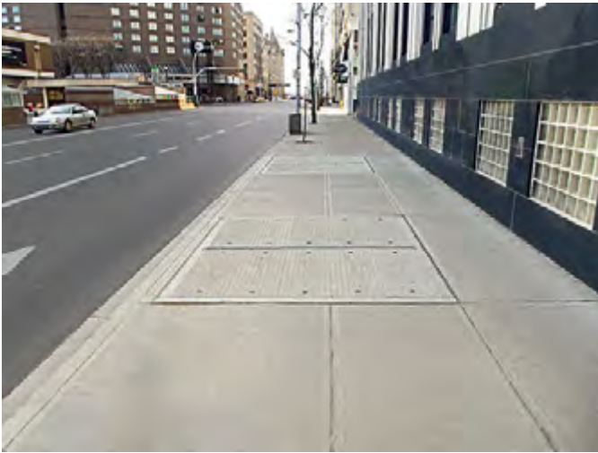
Finished cover installation in Edmonton
