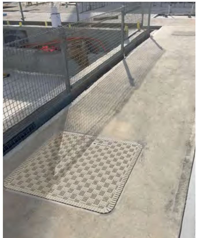
Installed cover over balance tanks
