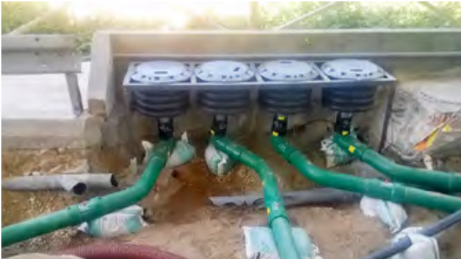
Cast iron chambers often have to be fixed in a frame and piping supported (pictured: different site to show possible frame configuration)
