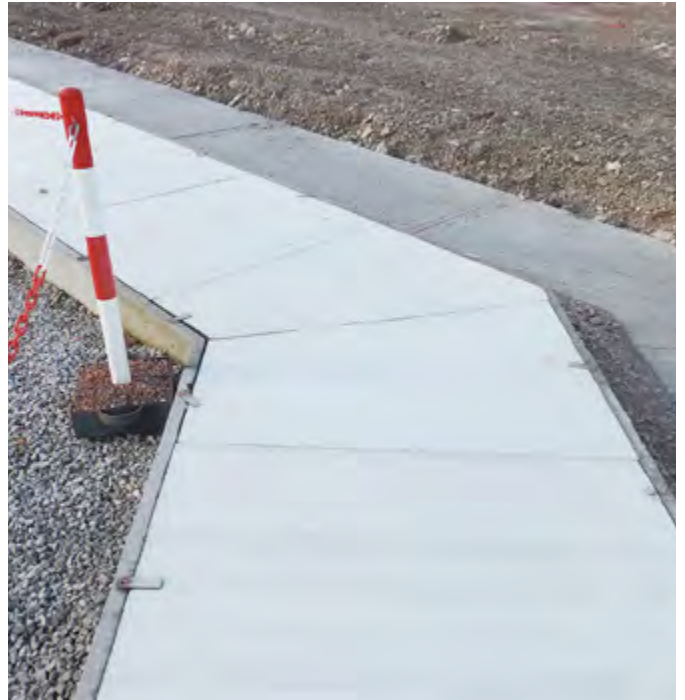
Previously installed low quality concrete covers
