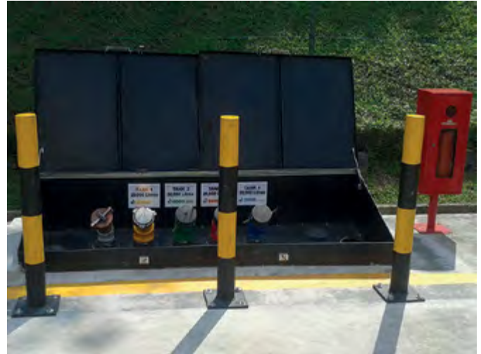
Fibrelite tank sumps being installed
