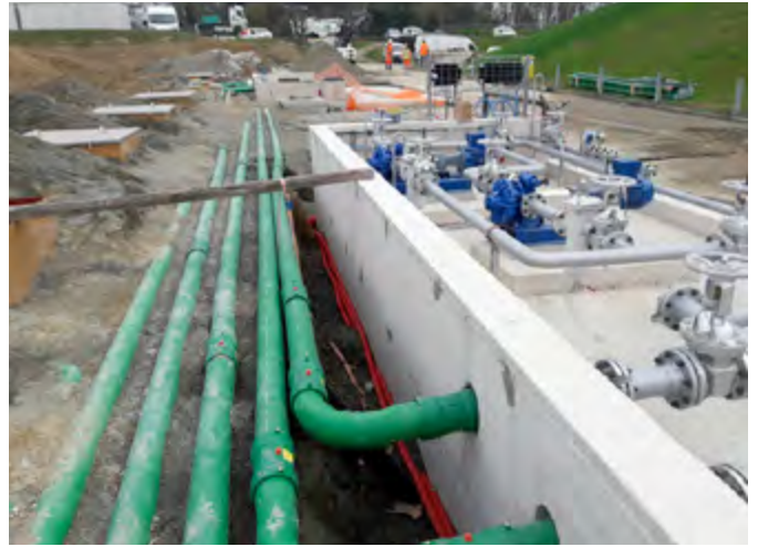
KPS conductive double wall piping provides the highest possible level of safety for Ethanol's potential to generate charge
