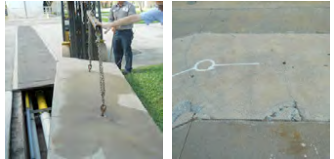
Traditional concrete panels are unsafe and labor intensive to remove and often break apart over time
