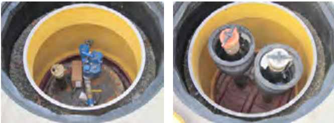
Fibrelite turbine and fill sumps
