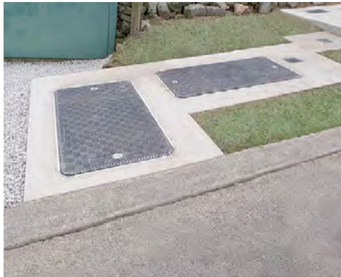
The 25 tonne load tested lightweight covers
