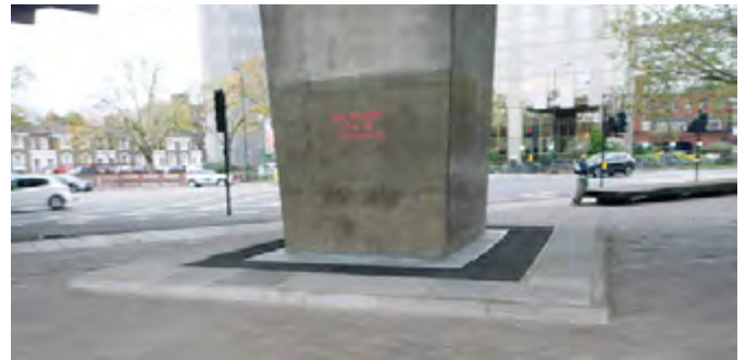
Roller bearings at the bases of supporting piers were replaced due to wear and increased load on the bridge
