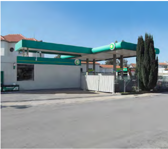
Site being upgraded with Fibrelite's fully conductive below ground remote fill sumps, covers and KPS conductive double wall fill pipe
