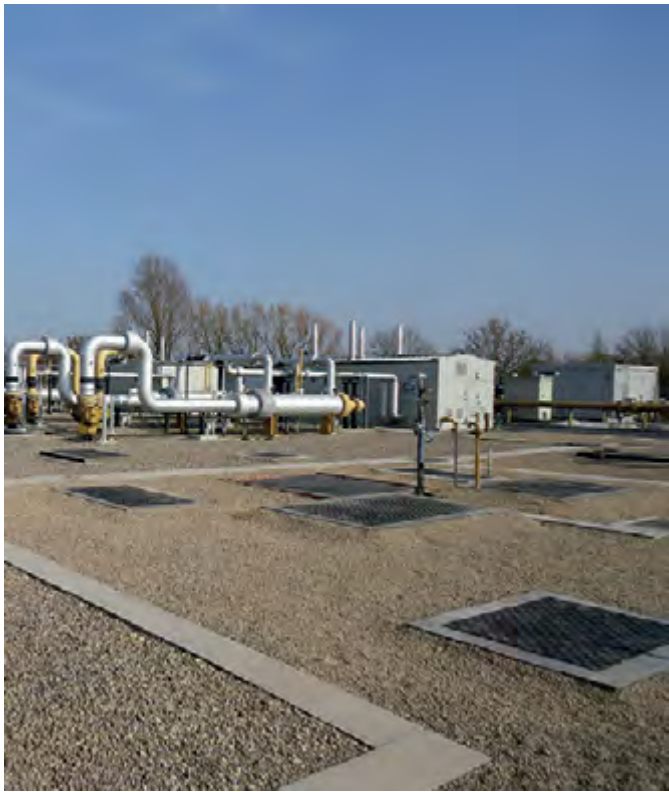
Fibrelite B125 (12.5 tonne) load rated lightweight trench and access covers
