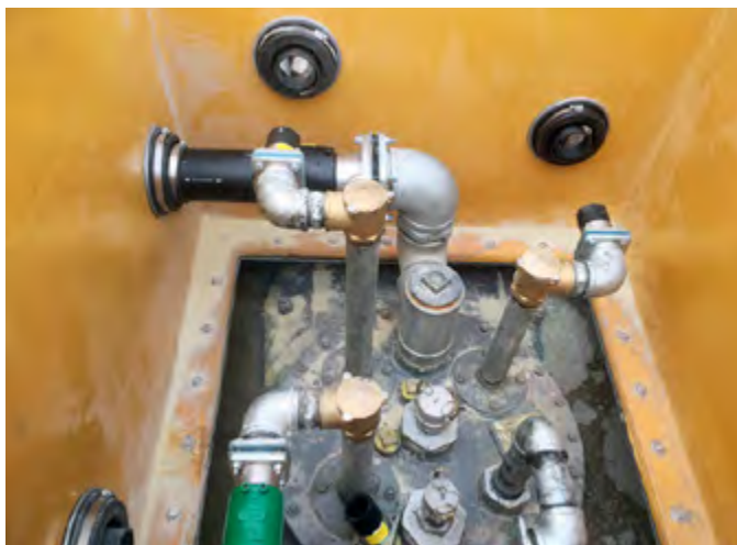
KPS piping, Fibrelite sumps and Fibrelite pipekits enable quick liquid-tight installations
