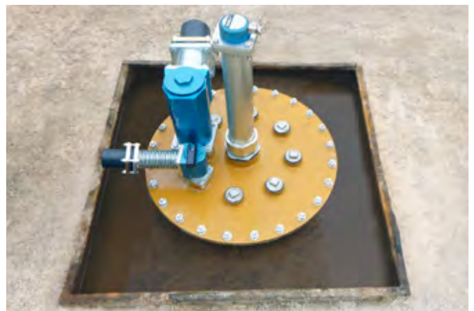
OPW's Fibrelite team came up with a solution to chemically bond the GRP square chambers onto the old tank upstands
