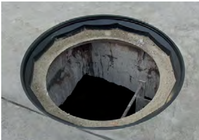
Fibrelite composite frame installed in sidewalk
