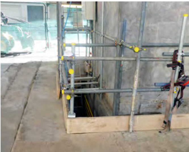
Spherical sliding bearings located in underground pits, allowing for minor movement of the pier
