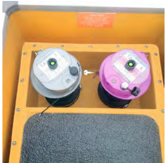
Factory fitted with dual contained KPS pipework for fills and single wall for stage 1 vapour line
