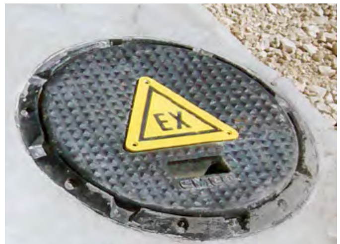
Previously used cast iron spill chamber
