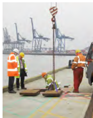
Costly and time consuming operation of removing the previously installed covers
