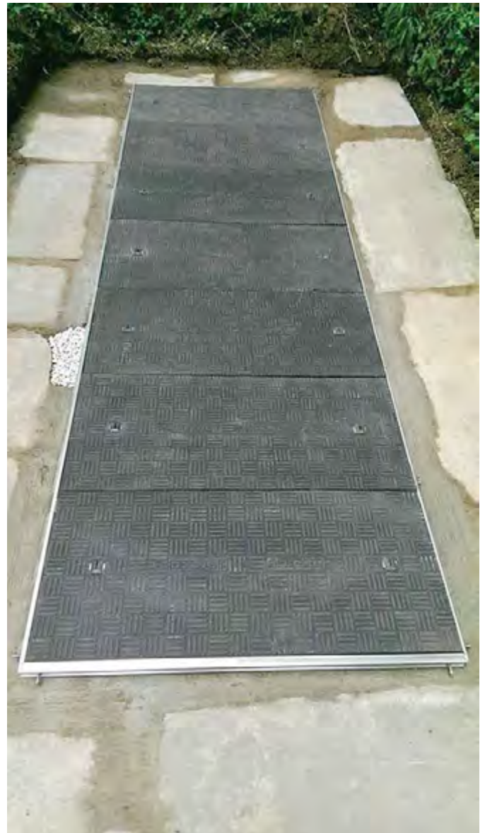
Chemically inert and corrosion resistant covers
