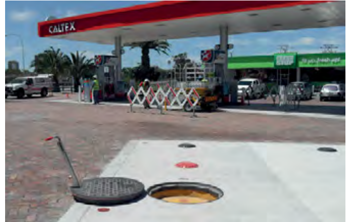
Watertight Fibrelite covers and tank sumps
