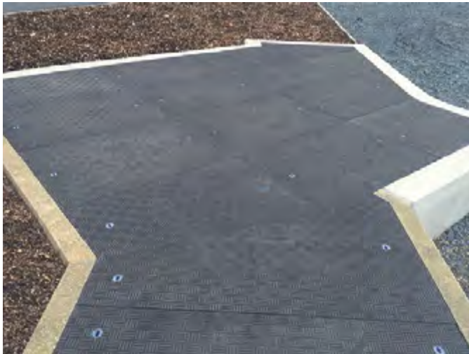
"Cassette" of bespoke covers over culvert
