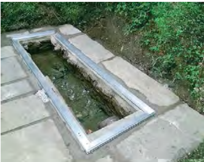
Fibrelite encapsulated frame
