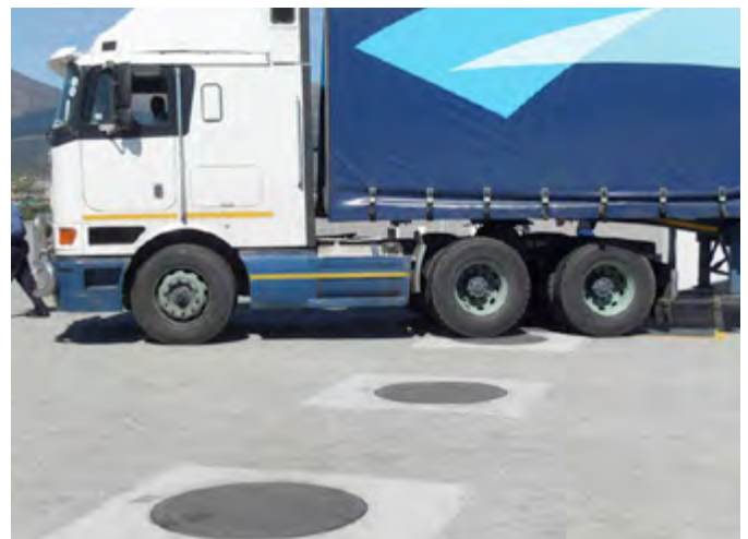
Fibrelite cover installed in truck lane
