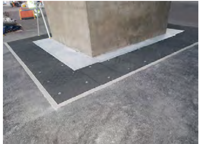
Replacement bearings located in the underground pits, covered by continuous set of access covers, allowing for the minor movement of the pier
