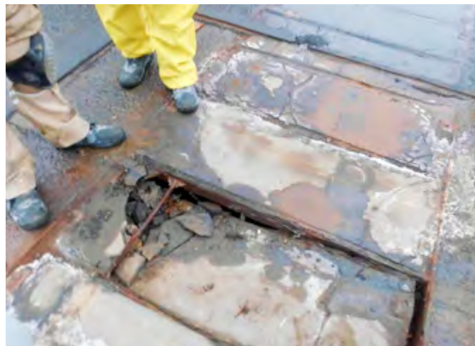
Heavily corroded previously installed covers
