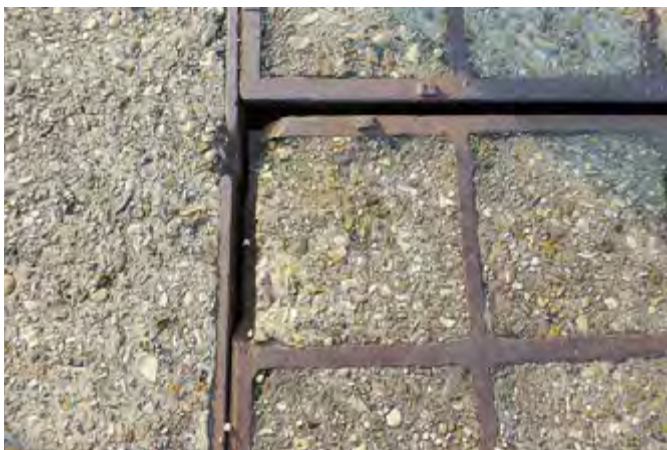
Corroding previously installed covers
