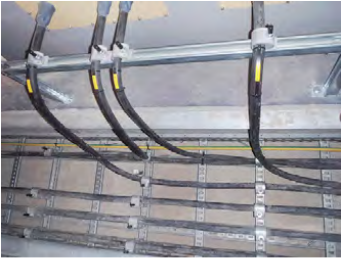
Expansive trench requiring coverage
