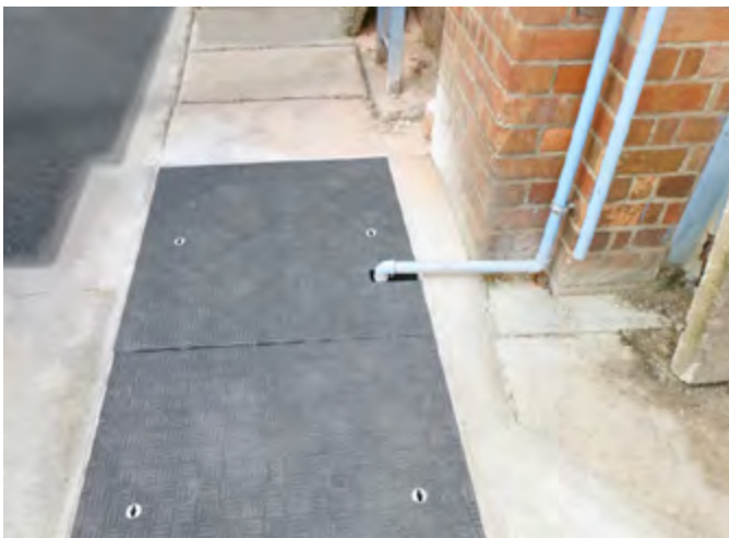
Fibrelite covers provide a lightweight alternative to concrete, alleviating health and safety risks
