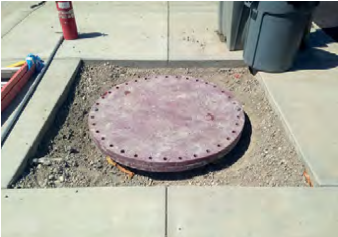
Fire protection tanks
