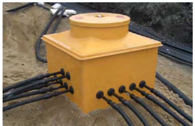
Fibrelite's electrical conduit drawpit being installed
