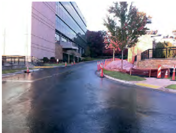
Pre-install location for the Fibrelite covers
