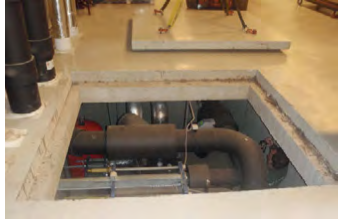
The geothermal monitoring pit
