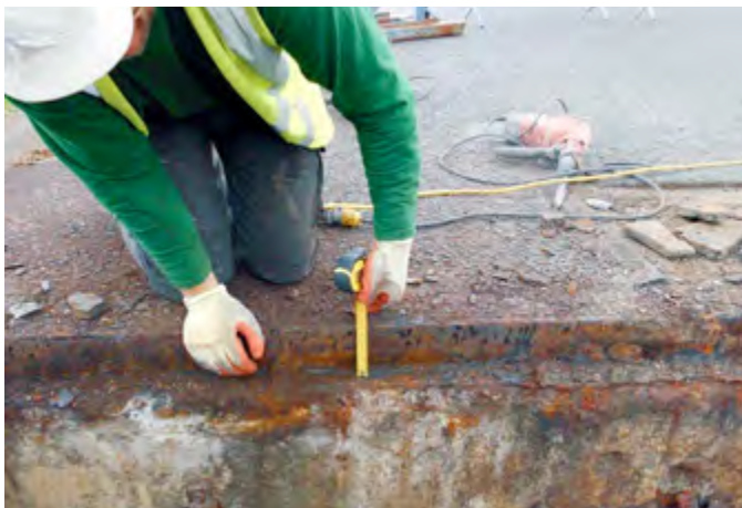
Previously installed heavily corroded access covers
