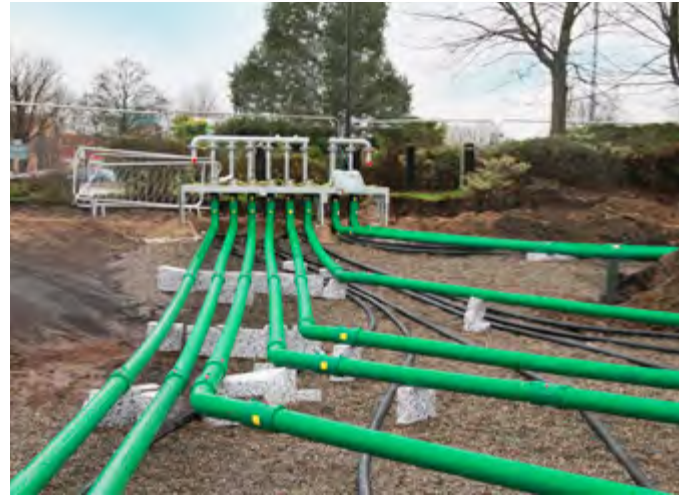
KPS formed bends below fill point
