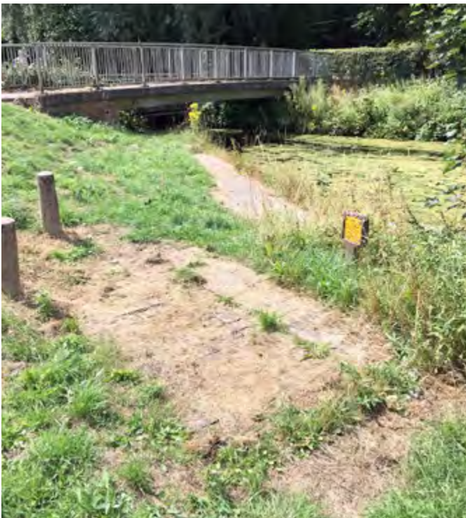
Previously installed covers had begun to degrade/rust
