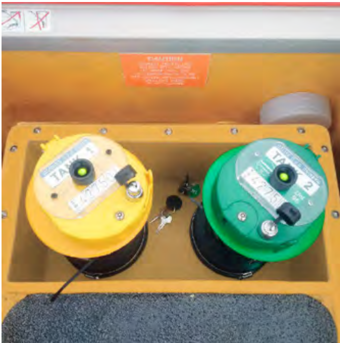
The fully conductive below ground remote fill systems are supplied with a non-slip working platform for the tanker driver to stand on
