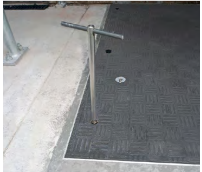
Secured/restrained covers, preventing unauthorised access
