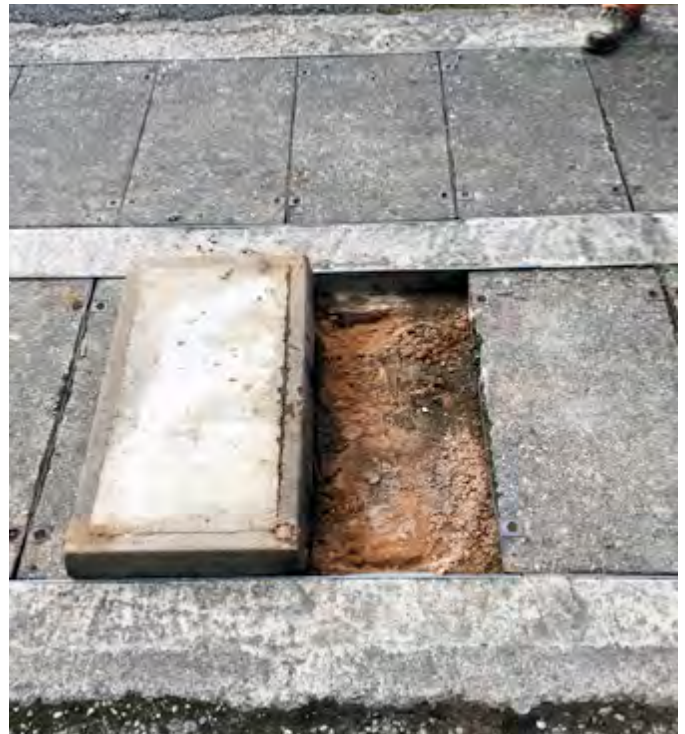
The previously installed covering arrangement was deteriorating
