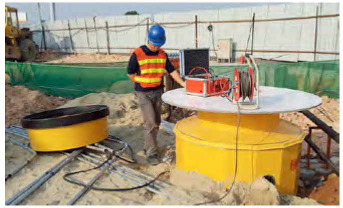
Vacuum tested tank sumps
