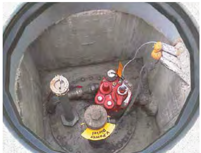
Fibrelite's covers prevented surface water ingress into chambers above the fuel tanks
