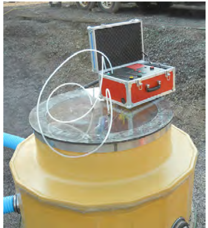
Vacuum testing to ensure a watertight installation
