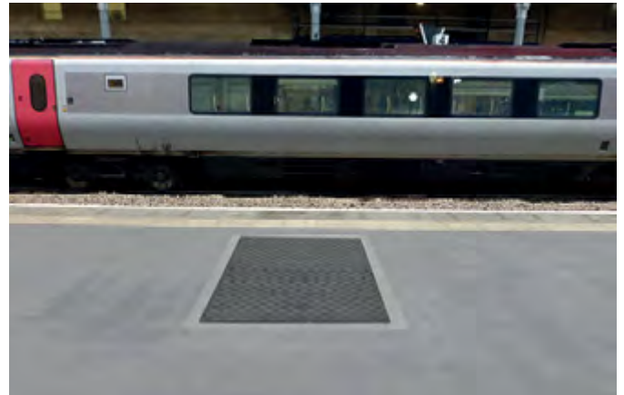
Lightweight Fibrelite covers now installed on platform
