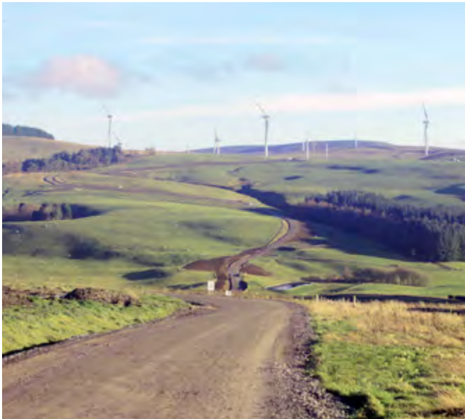
Garreg Lwyd wind farm under construction
