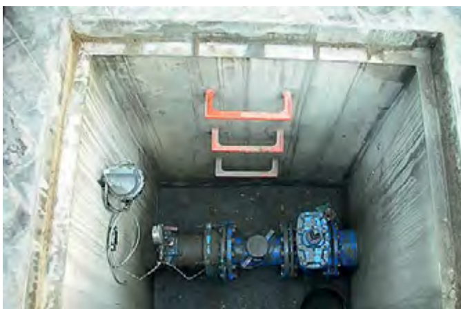
Automatic monitoring system located beneath metal cover which blocked signal (Image credit: Aguas de Cádiz)
