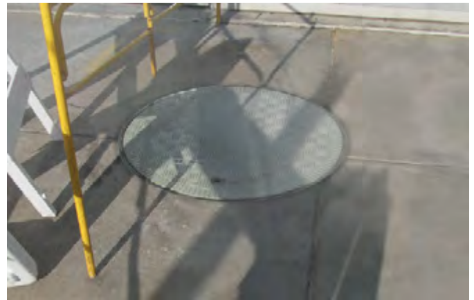
Fibrelite F95 composite cover installed in frame
