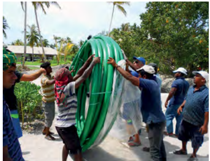
Unwrapping the KPS 75/63SCEC double wall fuel coil for the new fuel line
