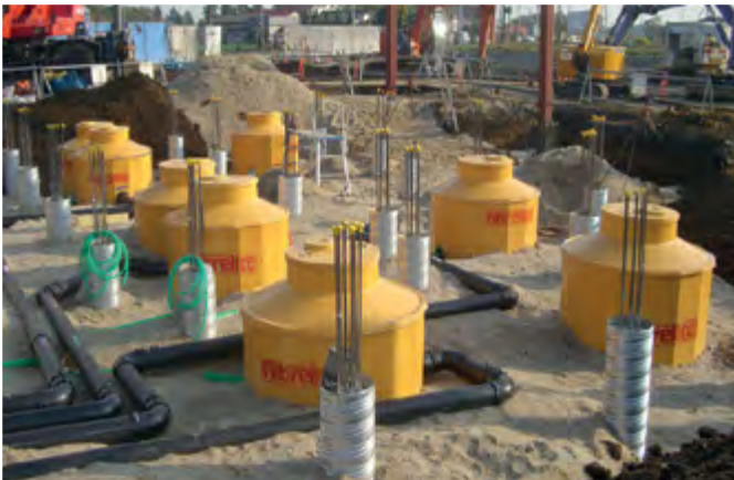
Fibrelite's 1.4m 16 sided tank sumps being installed
