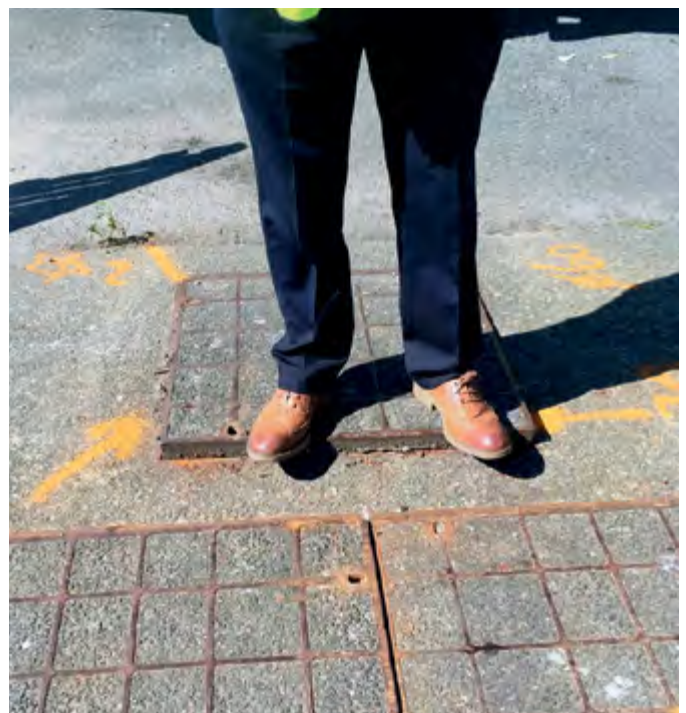
Previously installed heavy concrete recess covers were showing signs of severe corrosion
