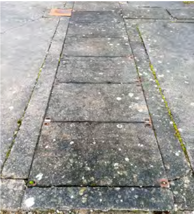
Previously installed concrete infill covers had deteriorated, making covers dangerous to remove, even with specialist personnel and equipment
