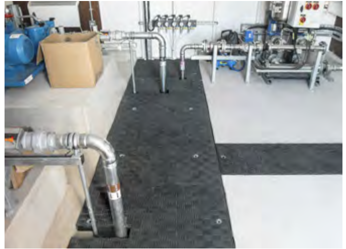
Fibrelite covers can accommodate service pipes of all shapes and sizes
