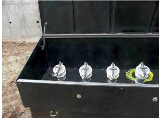
OPW heavy duty corrosion resistant seal caps
