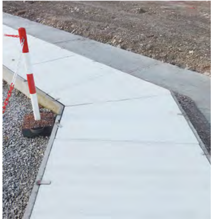
Previously installed low quality concrete covers
