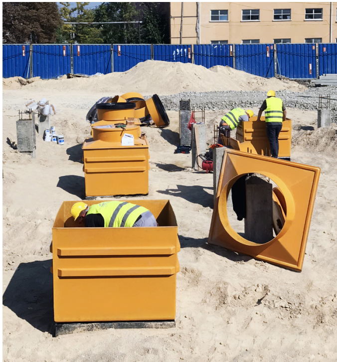
Technical support and installation training was required on site to complete the project within its tight timescale
